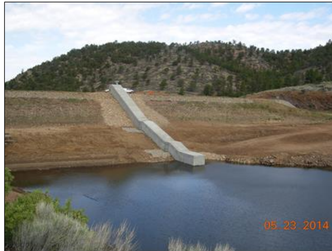
Nichols Dam Inclined Intake Structure. Reservoir Being Refilled. Photo 5/23/2014
