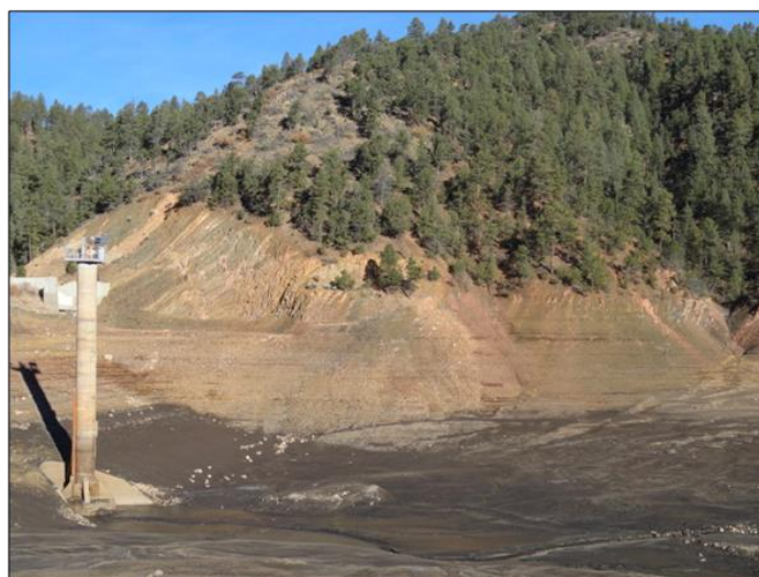
McClure Reservoir Fully Drained with Santa Fe River Flowing Directly Through Outlet. Photo 11/6/2014
