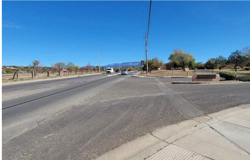
Figure 42: Camino de Chelly Access
