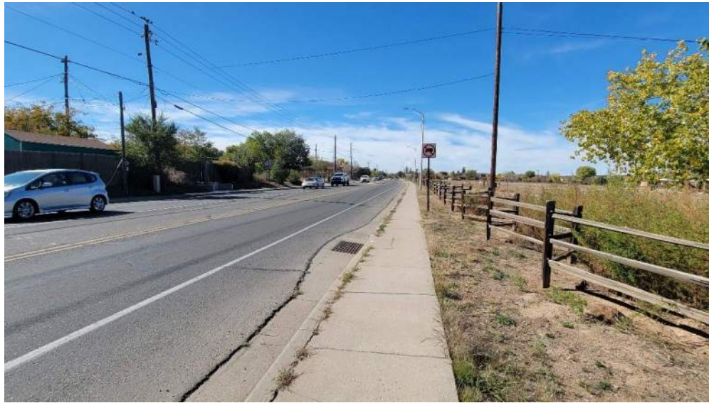
Figure 32: Drop Inlets in Bike Lane
