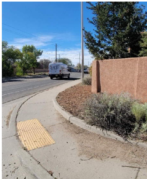
Figure 41: Ferguson Lane Sight Distance
