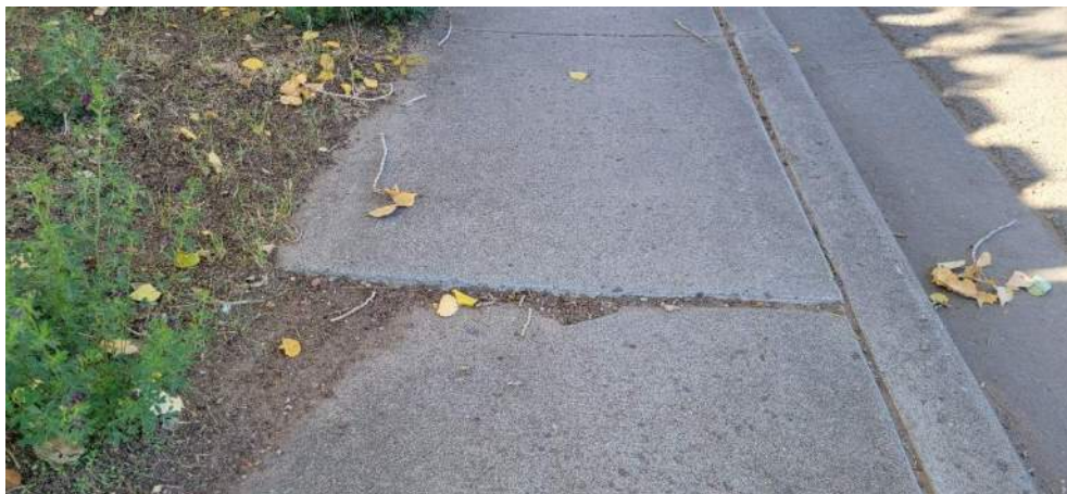
Figure 35: Uneven Sidewalk
