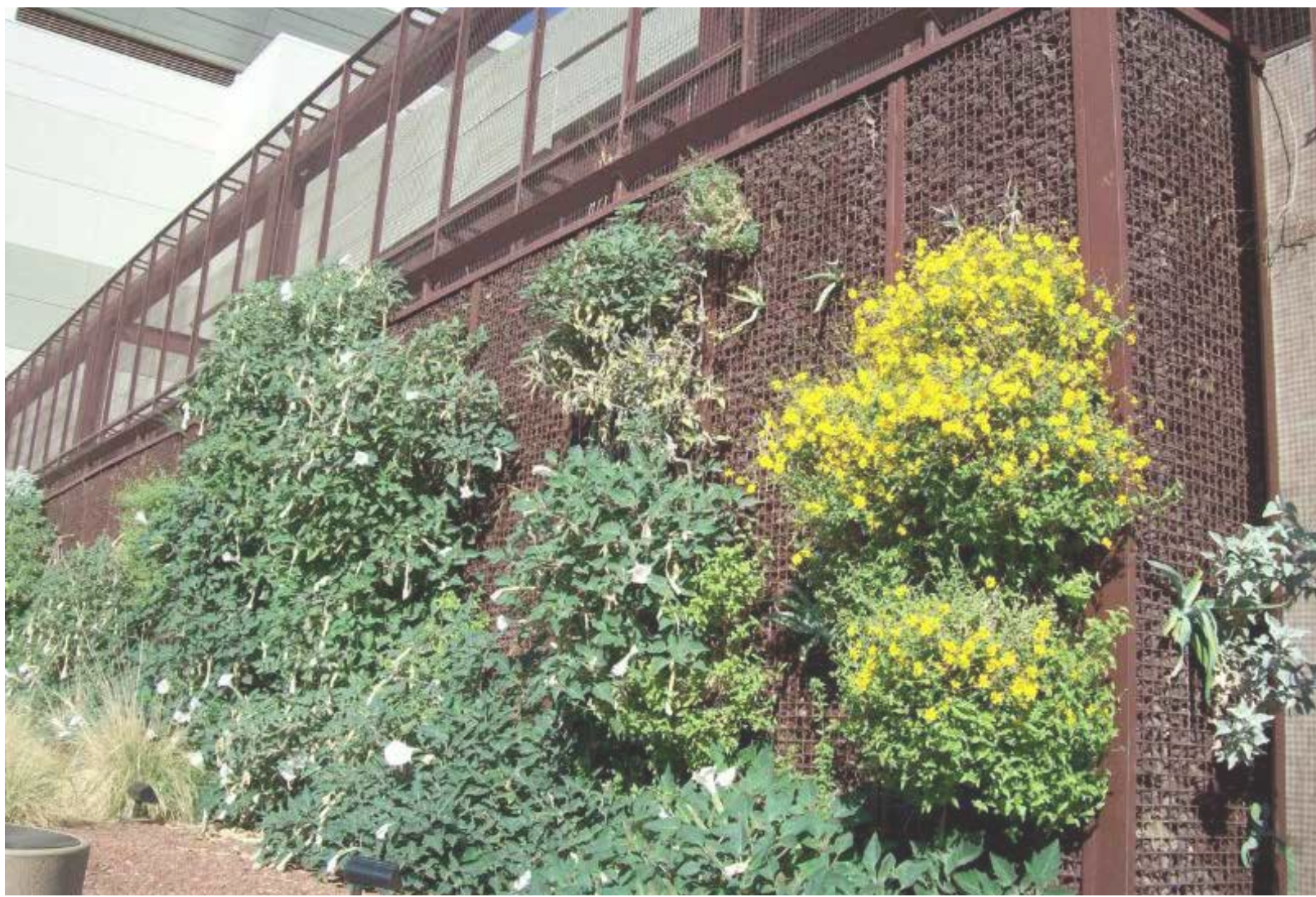
Seeded Gabion Retaining Walls
