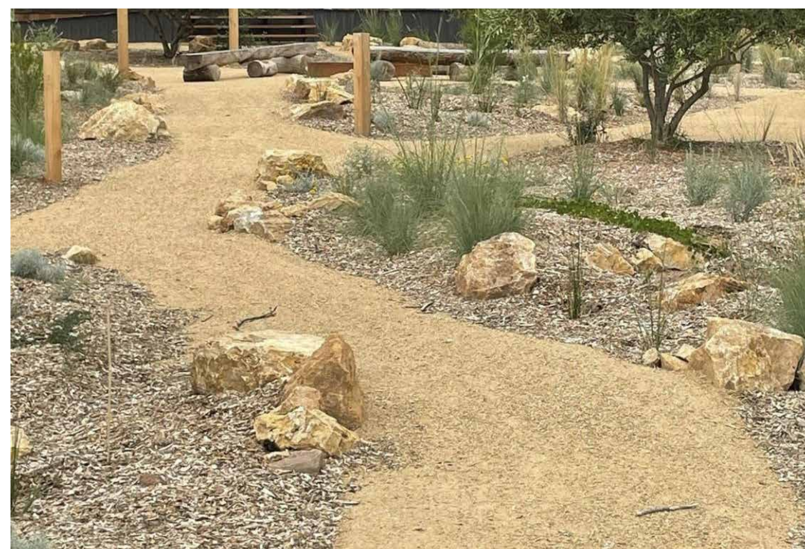
Crusher Fines Paving
