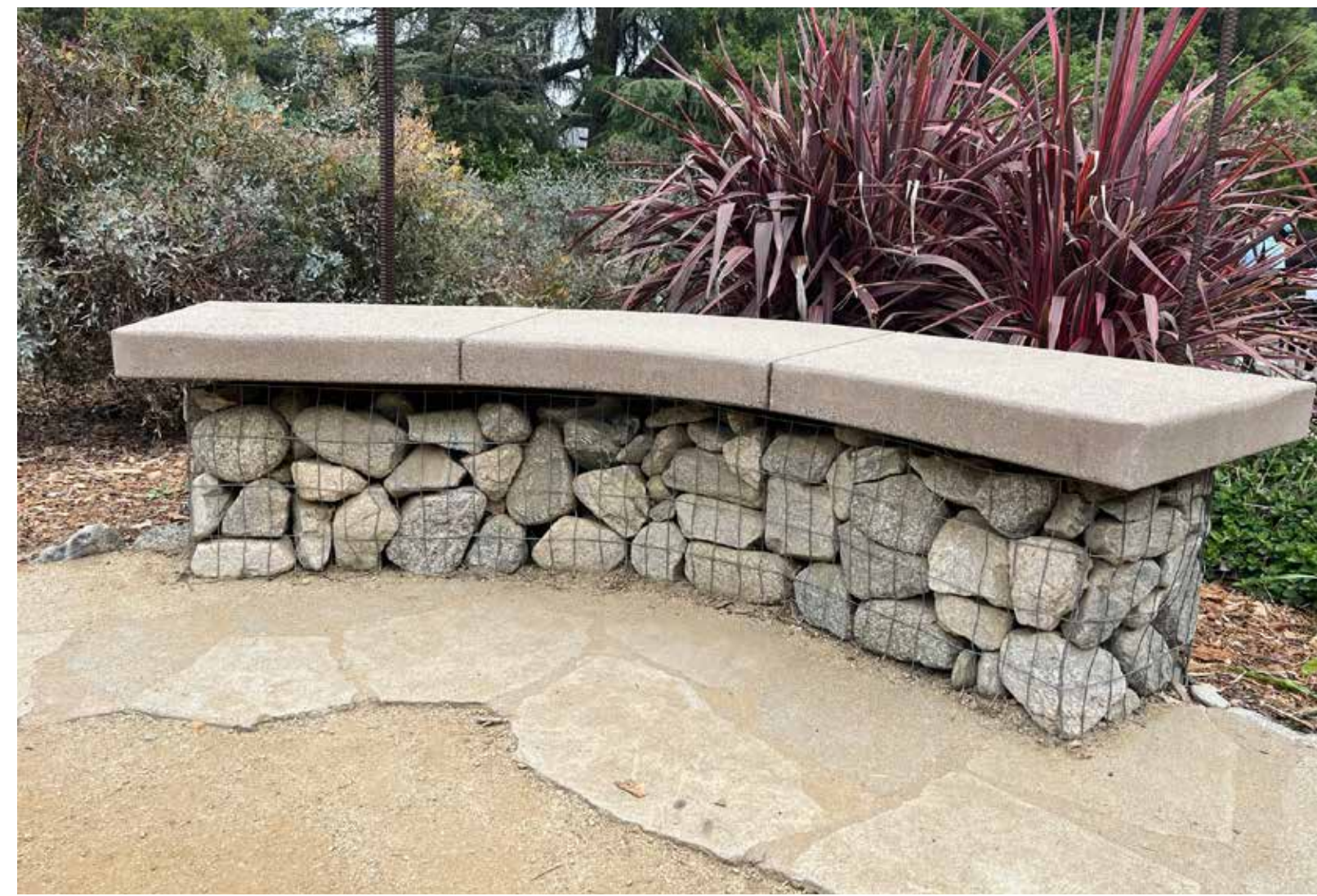
Gabion Seat Walls
