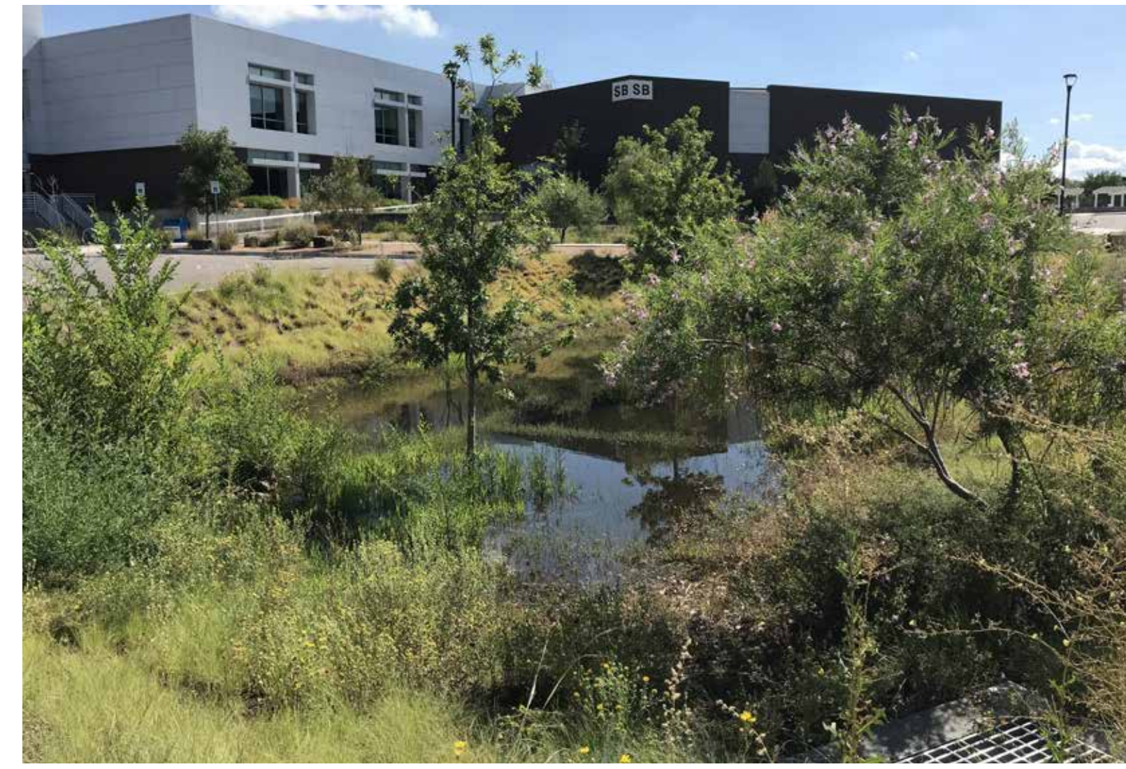
Stormwater Harvesting Basin
