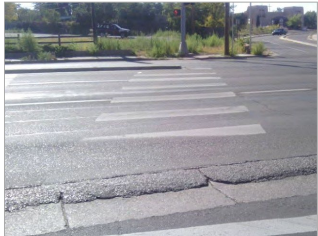
Figure 2-21: Median Obstructing Crosswalk
