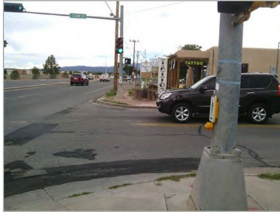
Figure 2-23: Missing Ramp and Sidewalk
