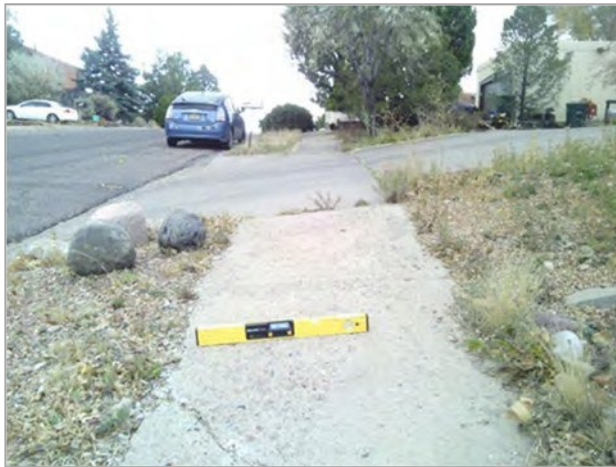
Figure 2-33: Non-Compliant Cross Slopes
