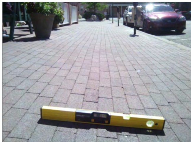
Figure 1-19: Example of a Steep Cross Slope
