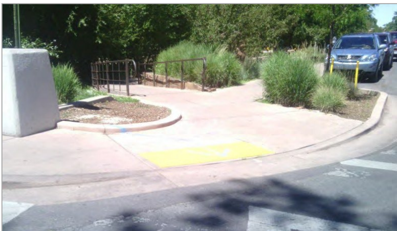
Figure 2-9: Curb Ramp without a Top Landing
