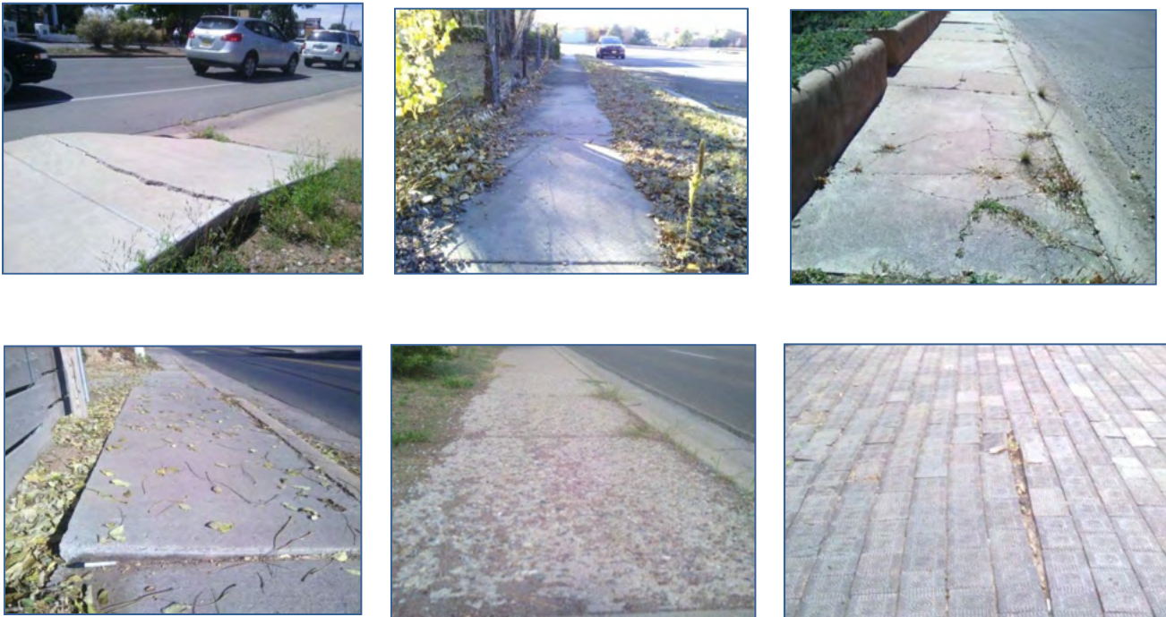
Figure 1-25: Examples of Surface Obstructions
