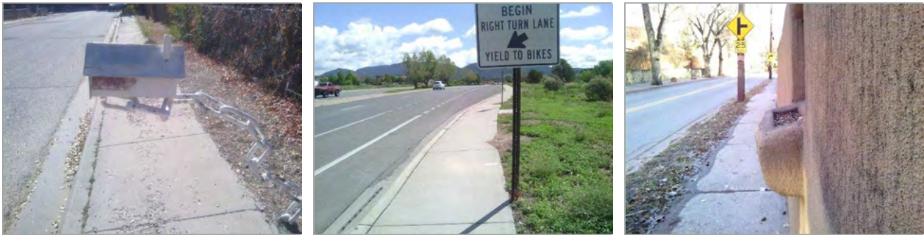
Figure 2-36: Sidewalk Protrusions
