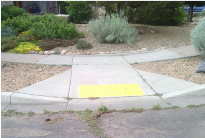
Figure 2-8: Curb Ramp with Non-Functional Flares
