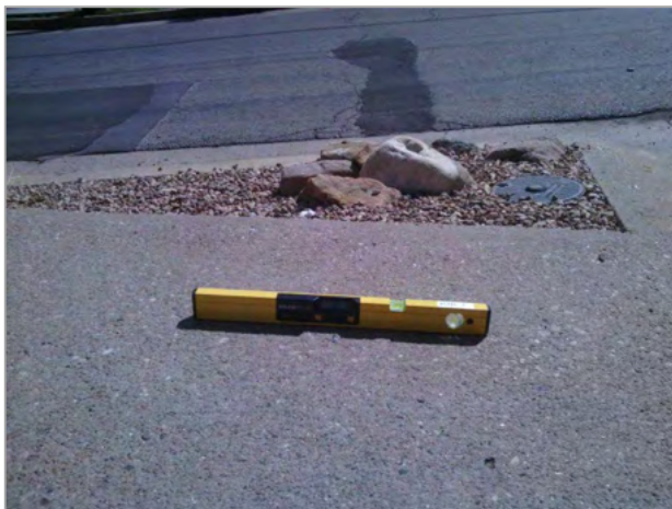
Figure 2-38: Non-Compliant Running Slopes
