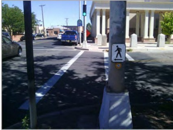
Figure 2-22: Missing Curb Ramp
