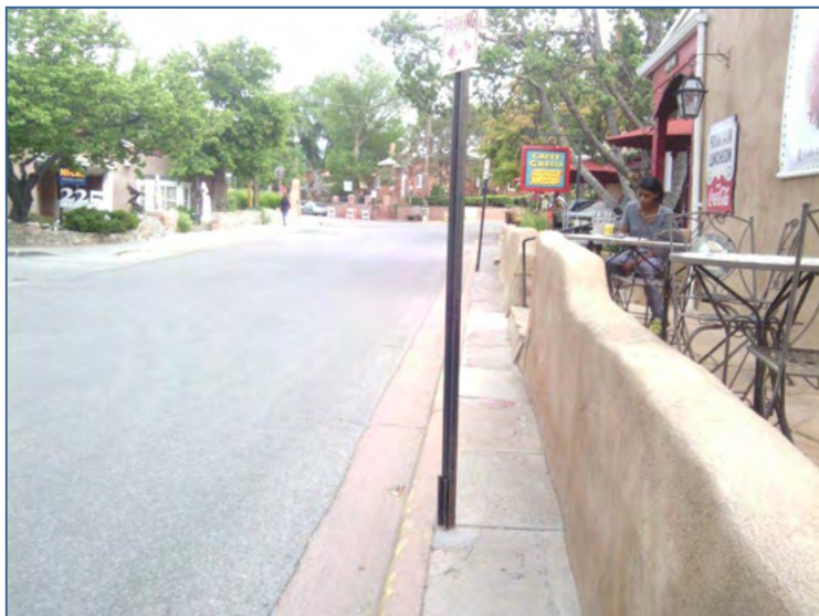
Figure 2-43: Less than 36-Inch-Wide Sidewalk
