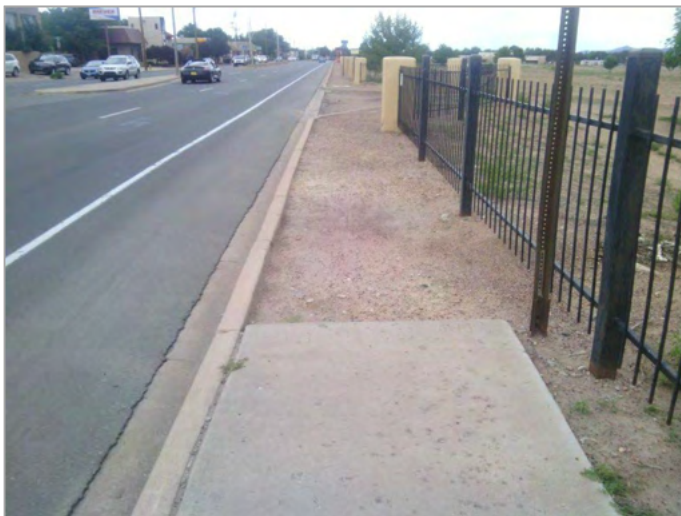
Figure 2-41 Non-Continuous Sidewalk Ends Mid-Block
