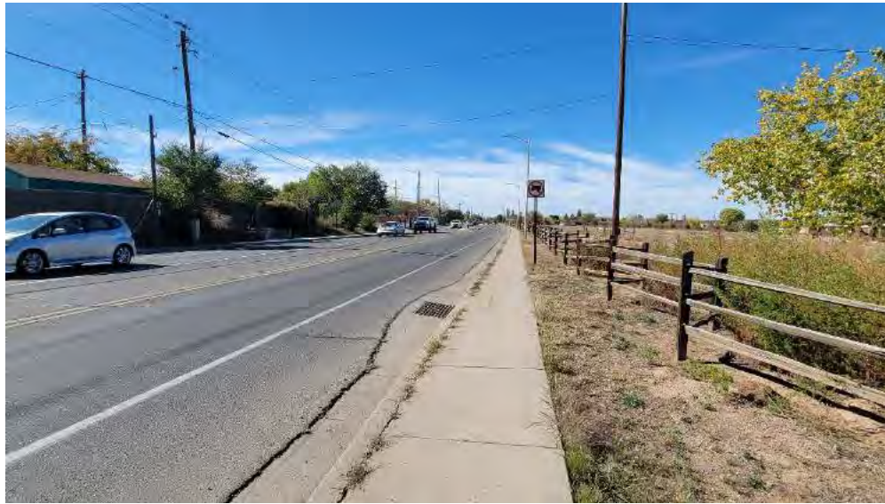
Figure 32: Drop Inlets in Bike Lane
