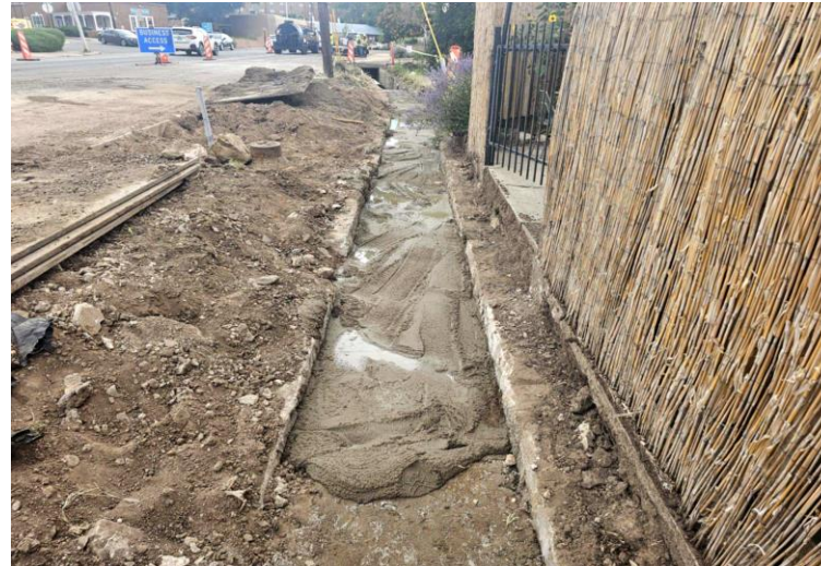
New concrete foundation
