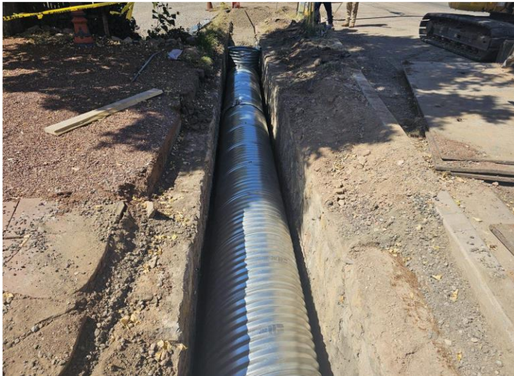
New storm water drainpipe
