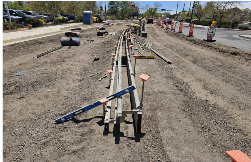
Concrete form placement for curb and gutter center median ST.16+25.
