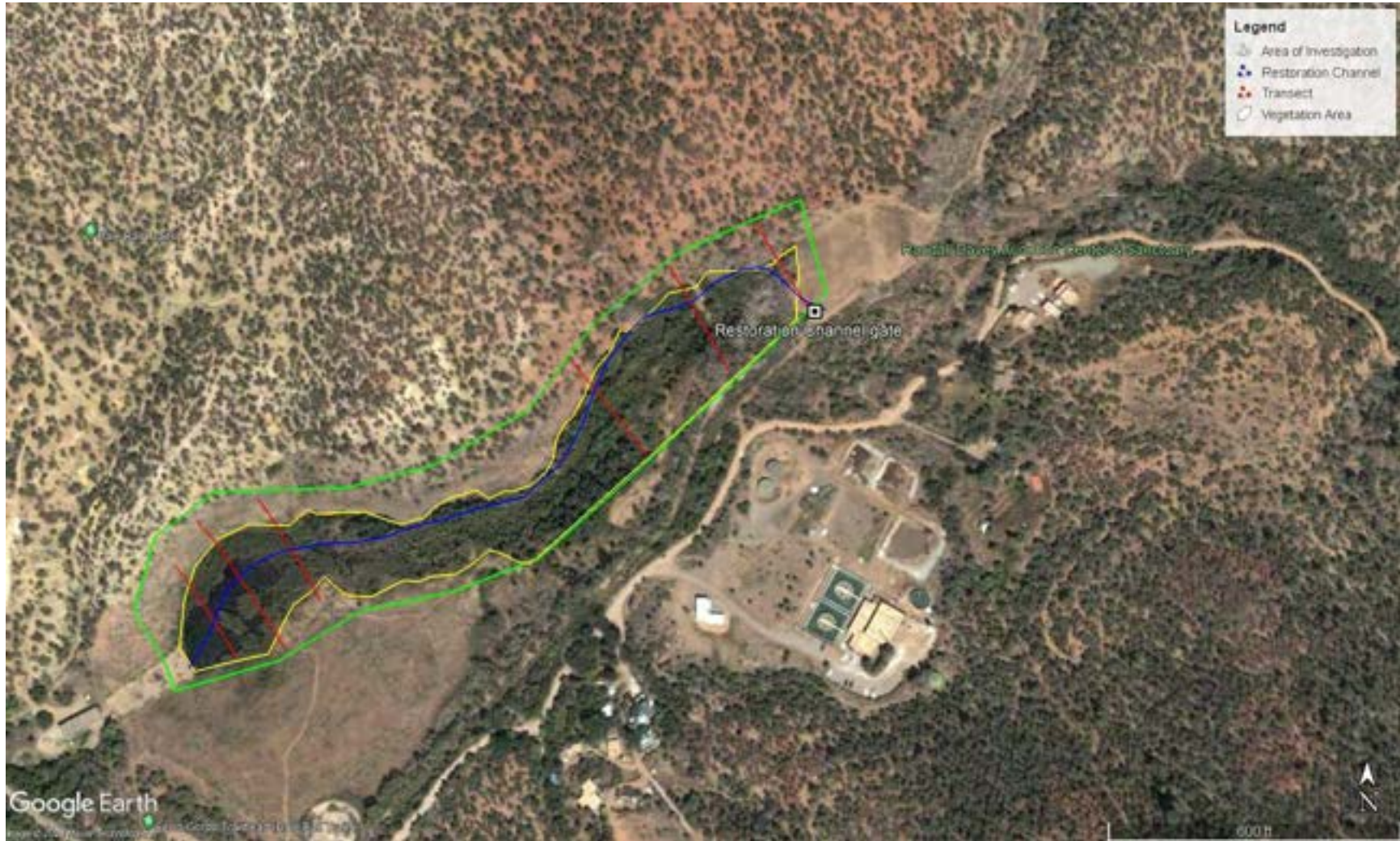
Figure A4. Historical image of Two-Mile Pond Complex dated May 10, 2004.
