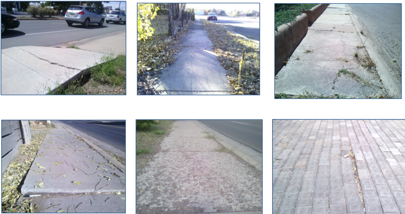
Figure 1-25: Examples of Surface Obstructions
