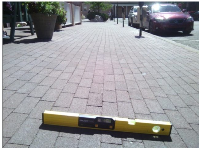
Figure 1-19: Example of a Steep Cross Slope
