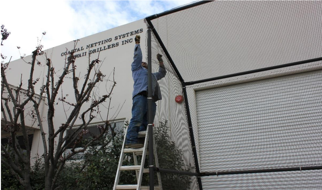
Step 12 – Attach Remaining Hose Clamps on All Spreaders & Legs @ 3' OC
