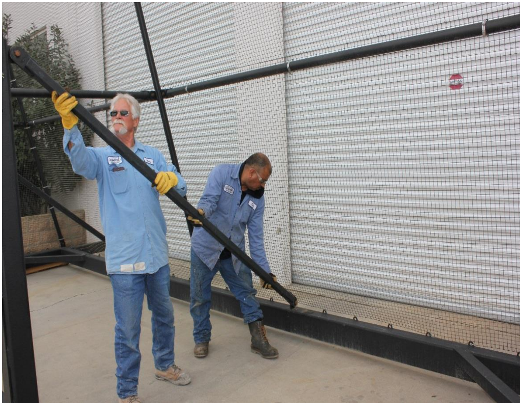
Step 15 – Attach Lift Unit Support Legs to Lift Unit & Base
