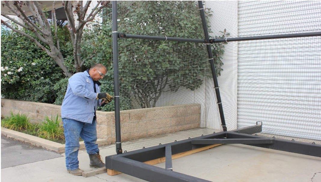
Step 12 – Attach Remaining Hose Clamps on All Spreaders & Legs @ 3' OC
