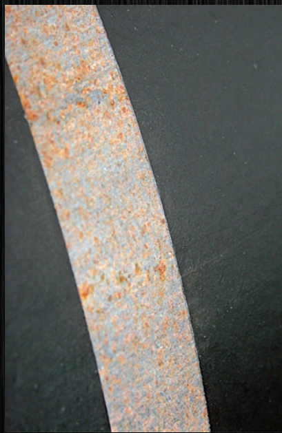
Three coats (10 mils applied on steel pole)
