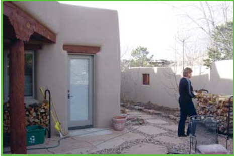
Move firewood away from structures.
