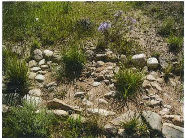
Open Channel Outfall – BMP – Infiltration Garden
