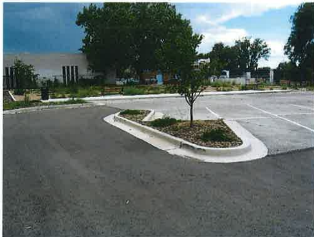
Porous Concrete Permanent BMP
