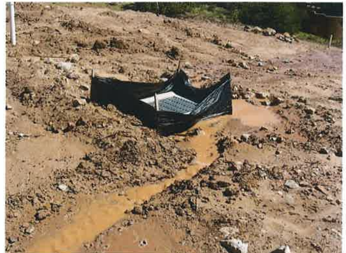
BMP - Inlet Basin Protection
