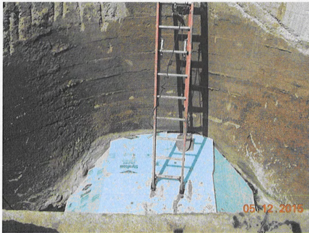
McClure Dam – Void Form Around Existing Outlet Conduit Prior to 1 st Concrete Pour May 12, 2015
