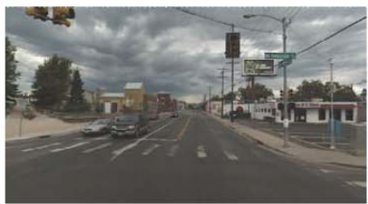
Two travel lanes in each direction, two-way center left-turn lane, attached sidewalks on both sides with utility poles
