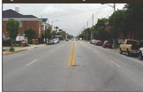
Figure 1. Photo. Four-lane configuration before road diet.
