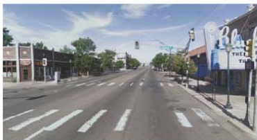
Two travel lanes in each direction, two-way center left-turn lane, on-street parking on both sides of the street, attached sidewalks with a tree and utility pole buffer on both sides.
