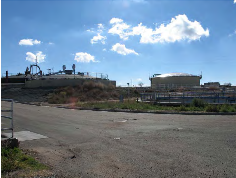
Figure 8-12. Existing Anaerobic Digesters and Sludge Holding Tank 2
