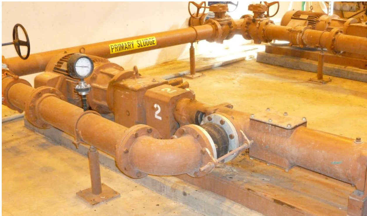
Figure 8-3. Picture of the Existing Primary Clarifiers (Top) and Sludge Pumps (Bottom)
