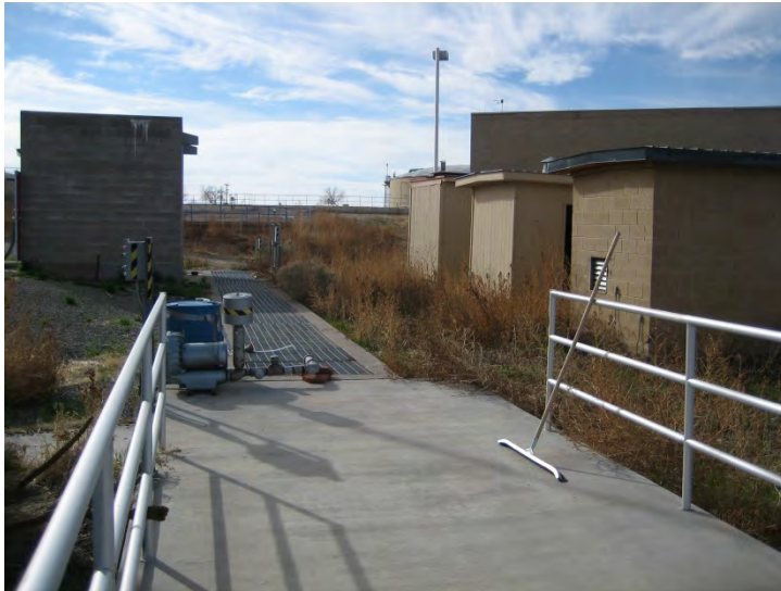
Figure 4. Reclaimed wastewater outfall channel and pump houses of users
