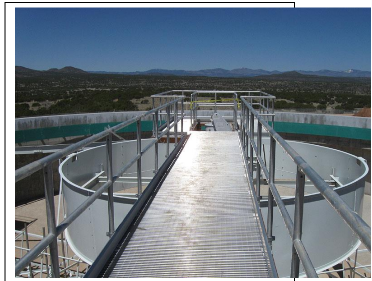
A view of the BDD gravity thickener.
