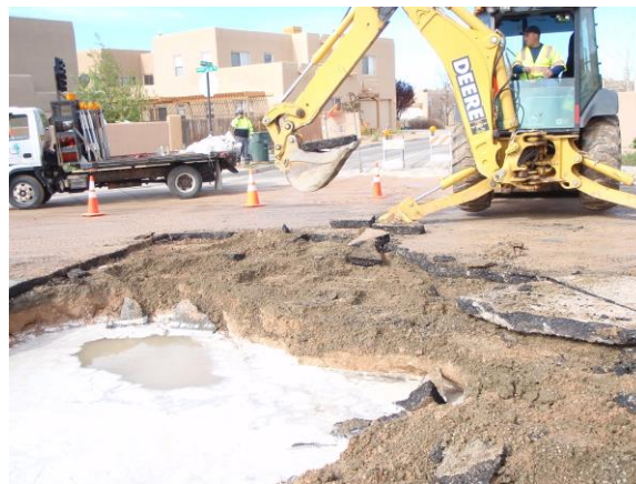
A member of the T&D staff repairs a main line leak.
