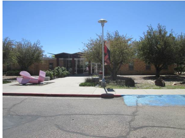
Administrative Building Front
