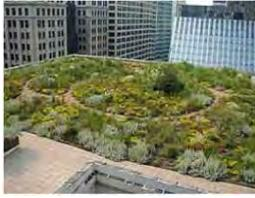
**Green Roofs** are another variation of a bio-retention cell that have a soil layer laying atop a special drainage mat material that conveys excess percolated rainfall off of the roof.
