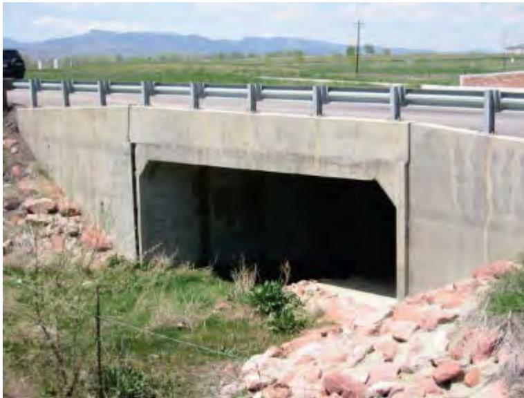
**Figure 3-2 Concrete Box Culvert**
