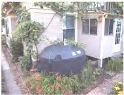
**Rain Barrels** (or **Cisterns**) are containers that collect roof runoff during storm events and can either release or re-use the rainwater during dry periods.
