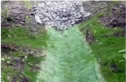
**Vegetative Swales** are channels or depressed areas with sloping sides covered with grass and other vegetation. They slow down the conveyance of collected runoff and allow it more time to infiltrate the native soil beneath it.
