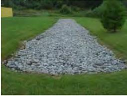
**Infiltration Trenches** are narrow ditches filled with gravel that intercept runoff from upslope impervious areas. They provide storage volume and additional time for captured runoff to infiltrate the native soil below.
