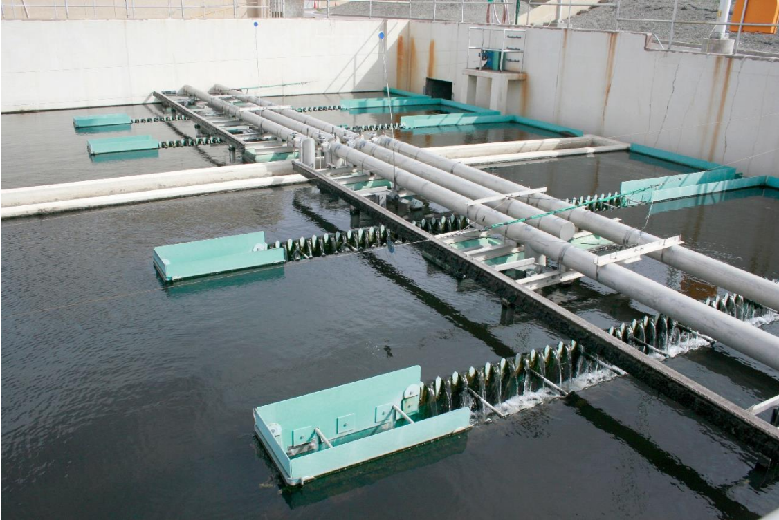
Figure 5: Secondary Clarifier Weirs and Clarivacs
