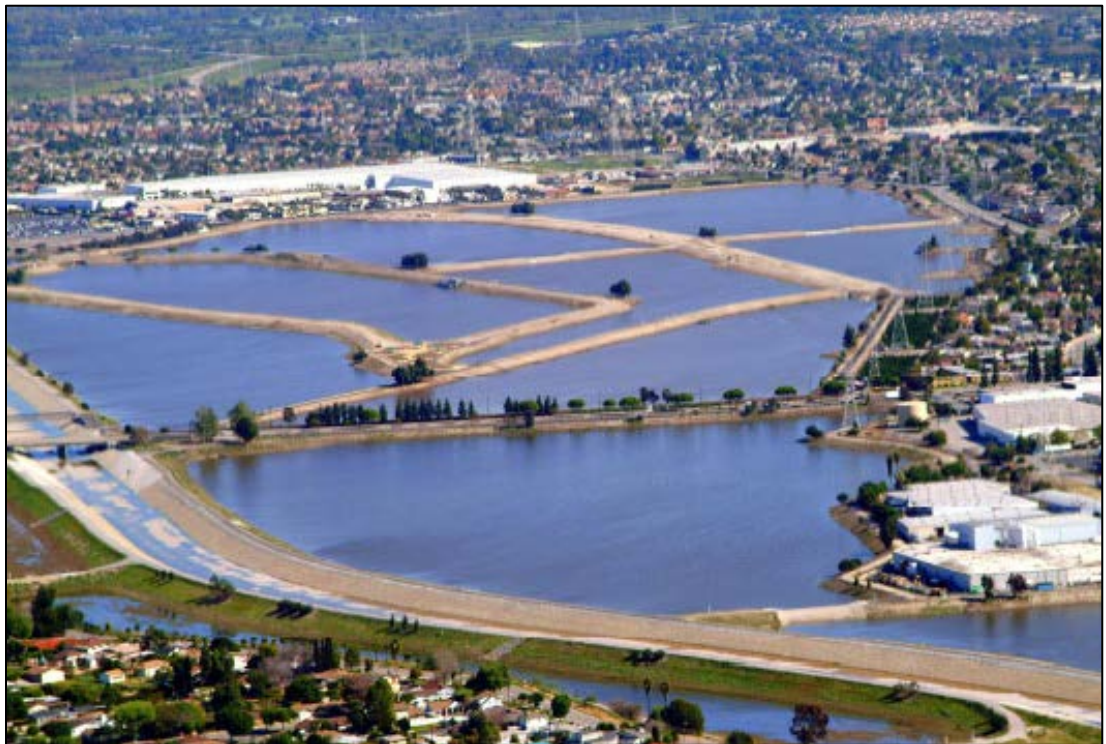
Rio Hondo Spreading Grounds
