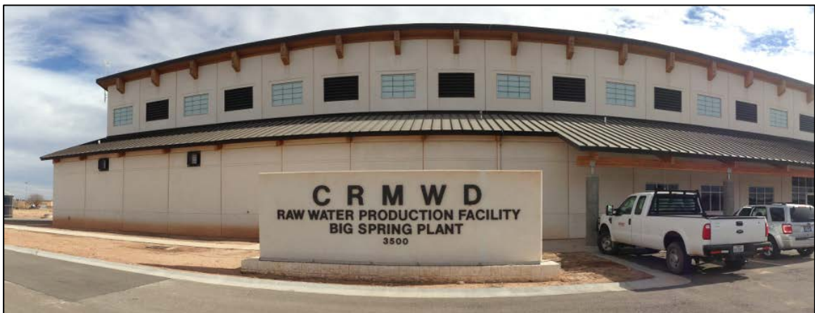
Colorado River Municipal Water District's Raw Water Production Facility in Big Spring, Texas
