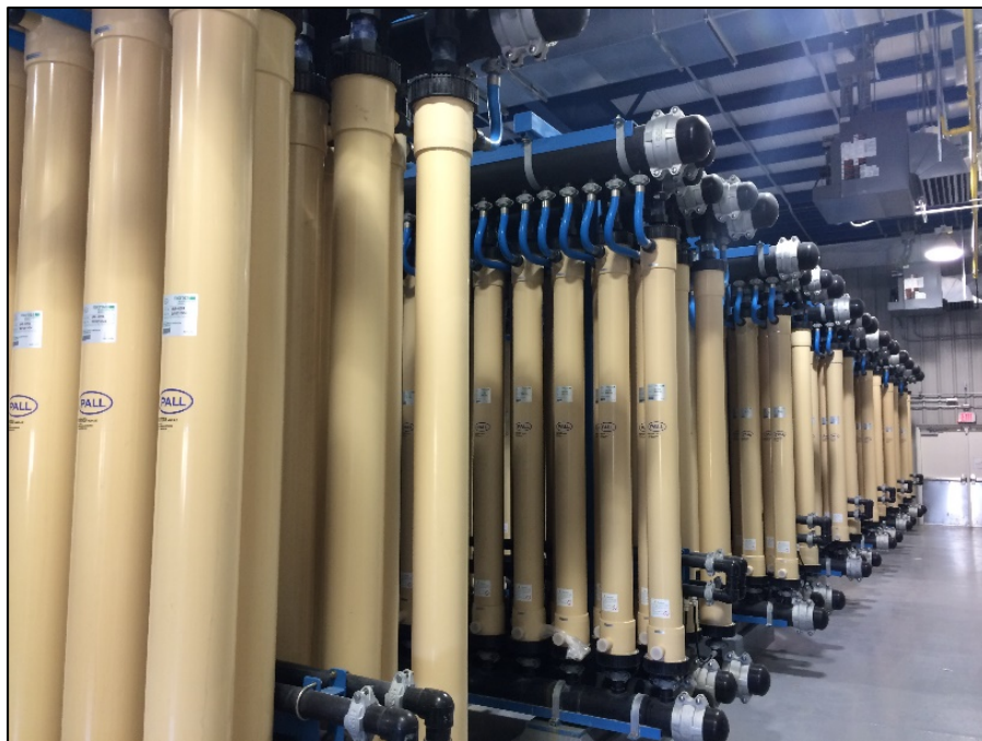
Reclaimed water from a new AWTF would be blended with Rio Grande water and treated at the BRWTF (shown here) under Alternative 7.
