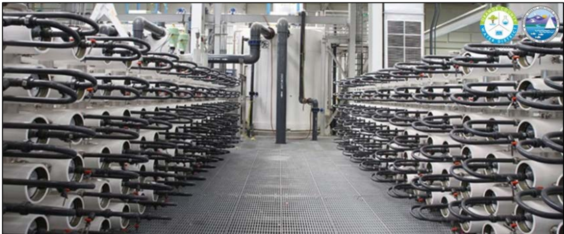
OCWD RO membranes used to purify reclaimed water for potable water reuse
