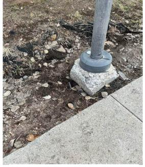
Photo 3: Exposed Footing for Existing Light Pole.
