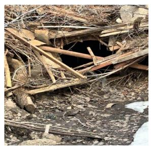
Photo 1: Partially Obstructed 48-inch outlet Pipe
