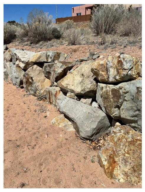
Photo 8: Boulder Retaining Wall on the north bank of Arroyo de Los Chamisos for embankment armoring
