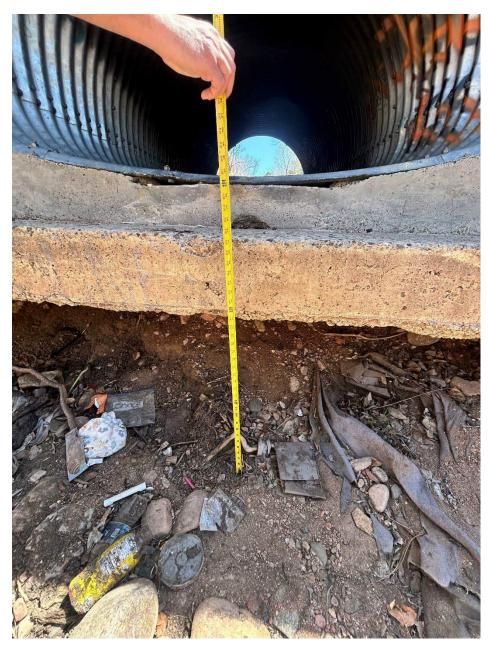
Photo 5: Approximately 3 ft difference between pipe invert and channel bottom
