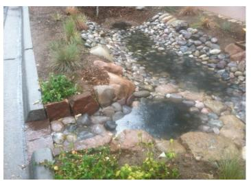
To capture pollutants and litter before they enter the Santa Fe River To encourage infiltration to support adjacent plant life To reduce the damaging, eroding forces of storm water
