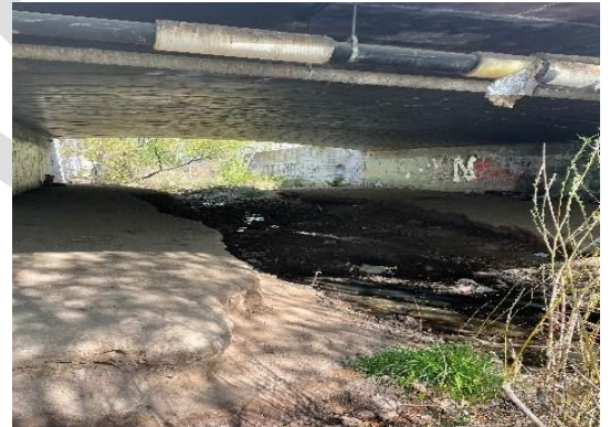
Sandoval underpass after cleanup
