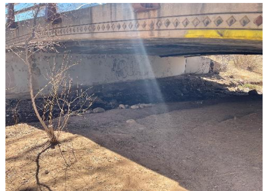
Paseo de Peralta underpass after cleanup
