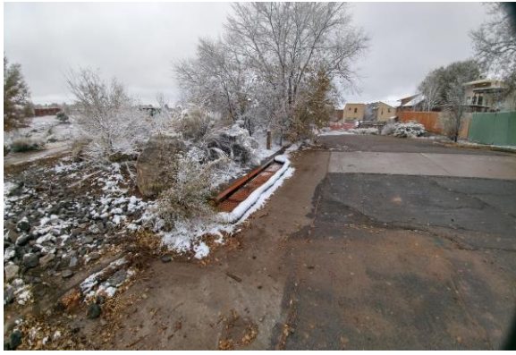
Photos 2 & 3: Protect Storm Drain and Track Pad Entrance
