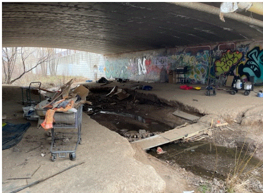
Sandoval underpass before cleanup
