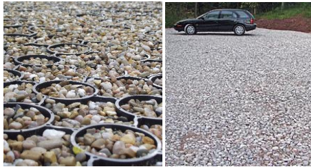
Rural example of permeable pavement (1)
