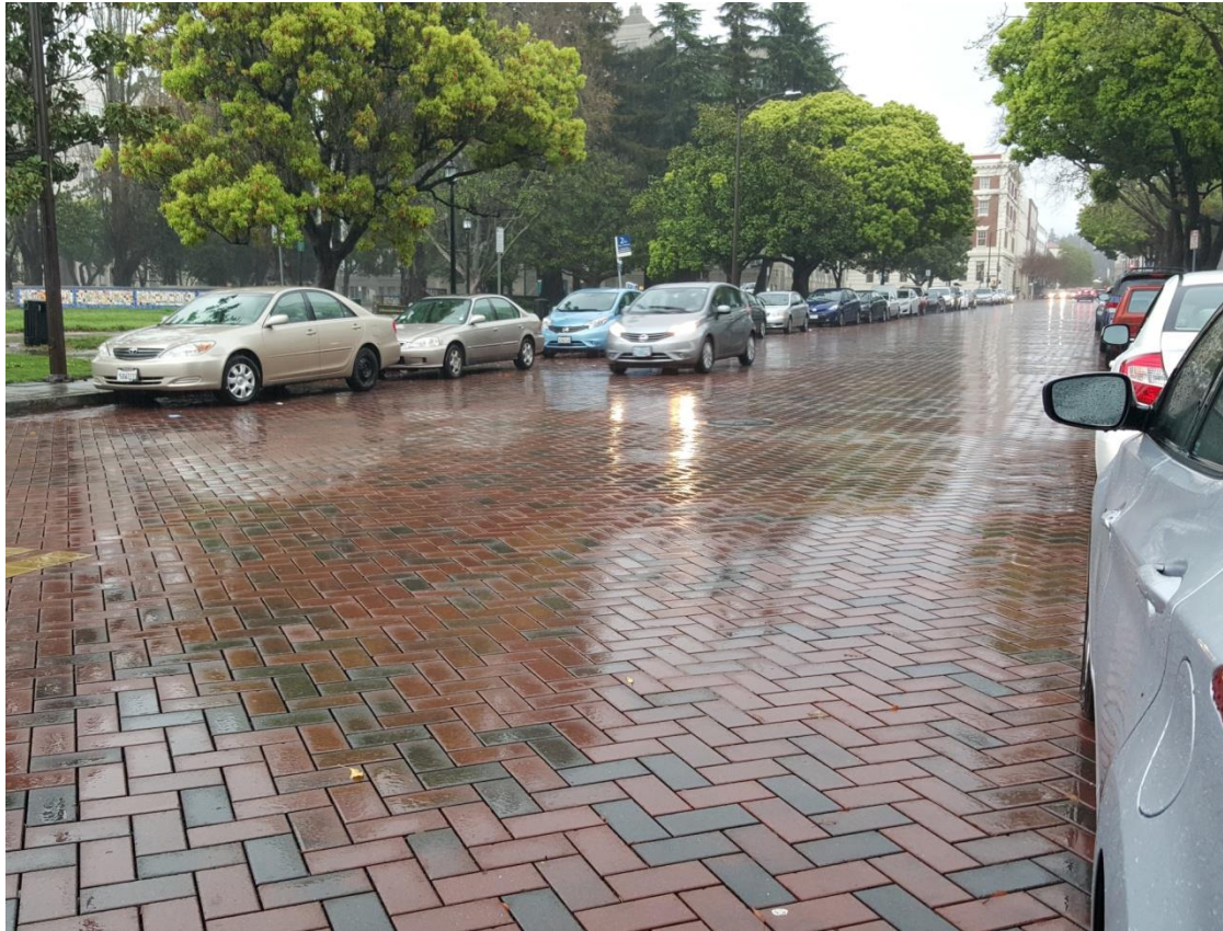
Allston Way in Berkeley, California was completely renovated with permeable interlocking concrete pavers. (Photo Source: https://www.cleanwaterprogram.org/index.php/programs/green-infrastructure/greenstreets-examples.html )
