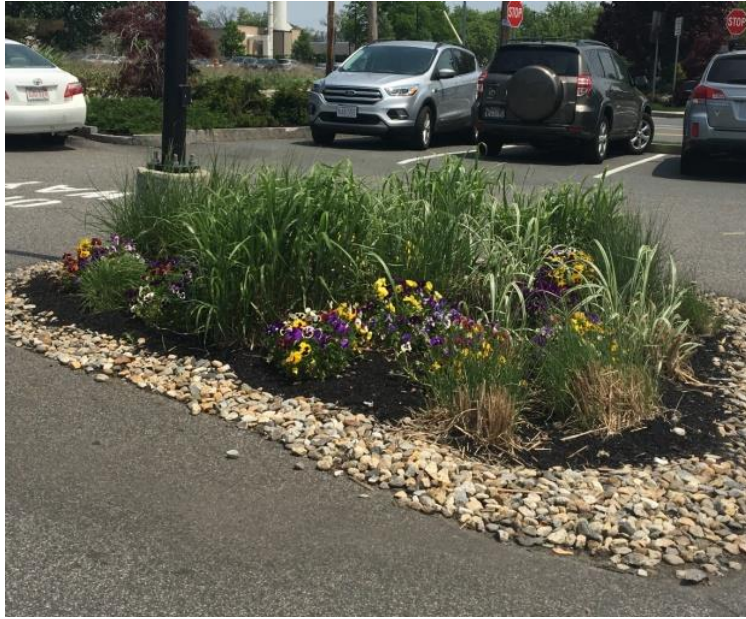
Example of Removal of Impervious Surface (1)
