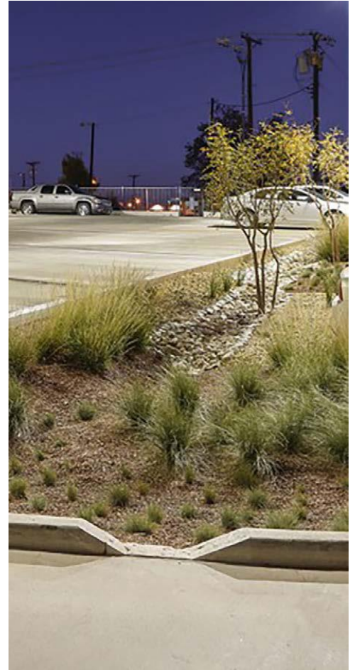
Example of a bioswale with bioretention/bioinfiltration taking stormwater from a parking Lot (2)
