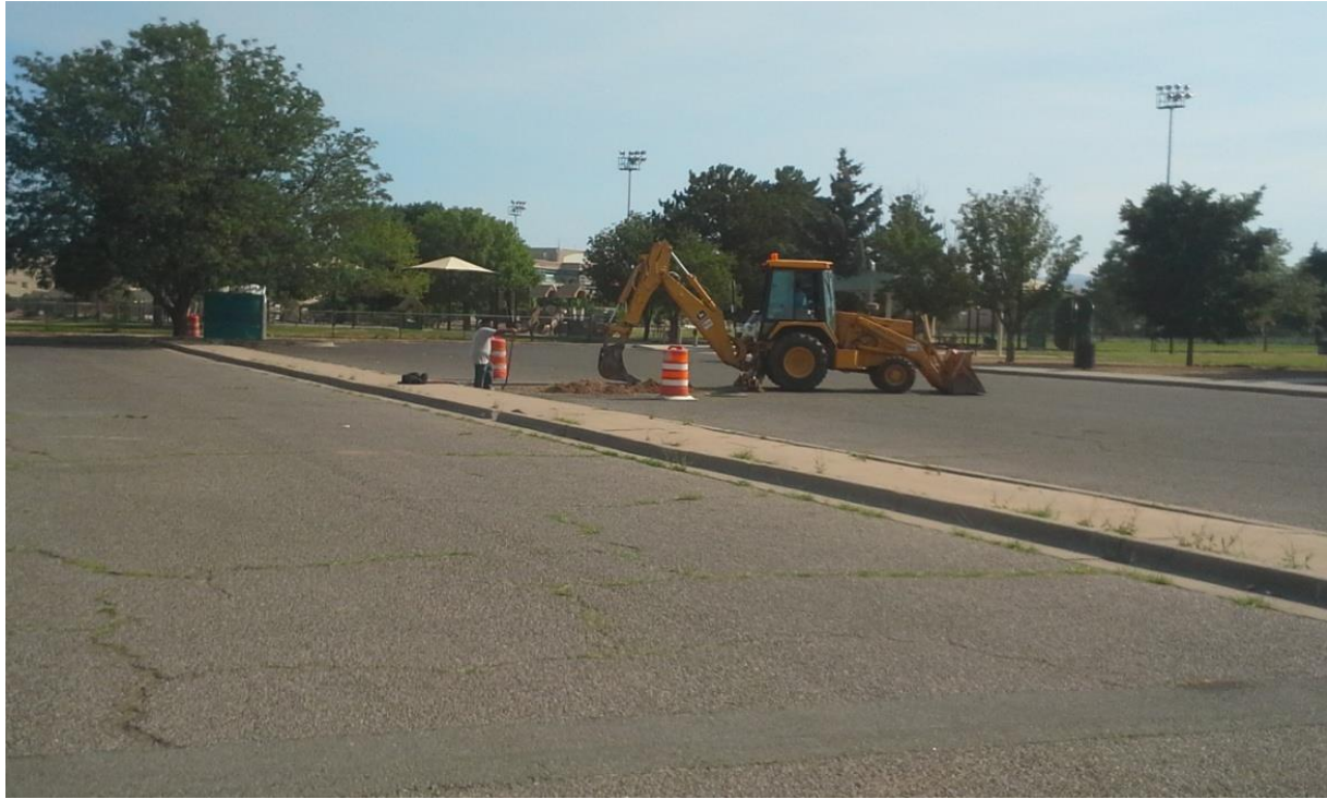
Pavement from underutilized parking spaces being removed in General Miles Park and replaced with rain gardens to promote infiltration. (Photo credit: Santa Fe Watershed Association)
