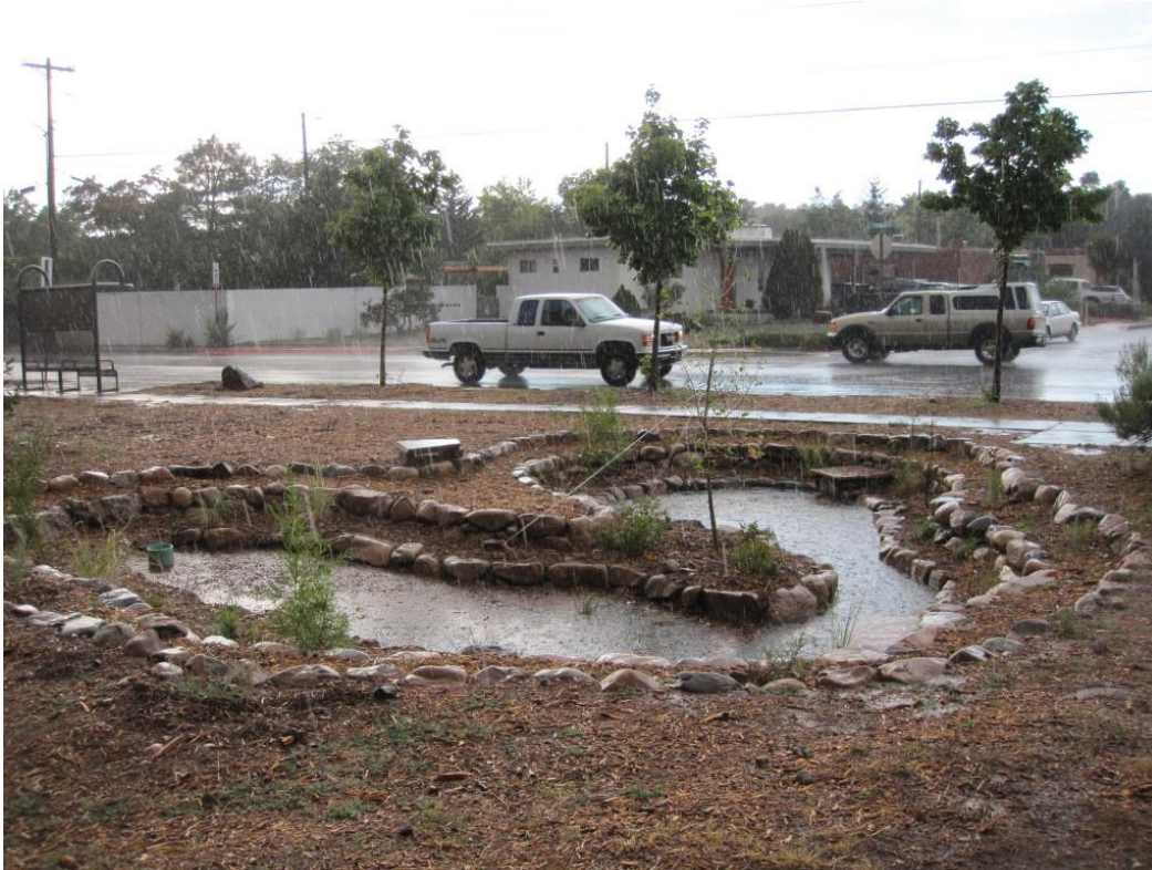
A small bioretention system was constructed in 2016 by retrofitting an existing vacant curb median at the intersection of Espinacitas and Hopewell streets in Santa Fe. (Photo credit: Santa Fe Watershed Association).
