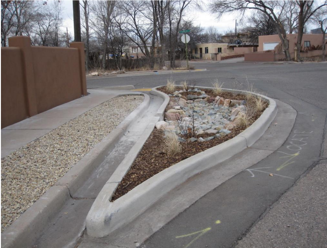
A small bioretention system was constructed in 2016 by retrofitting an existing vacant curb median at the intersection of Espinacitas and Hopewell streets in Santa Fe. (Photo credit: Santa Fe Watershed Association).
