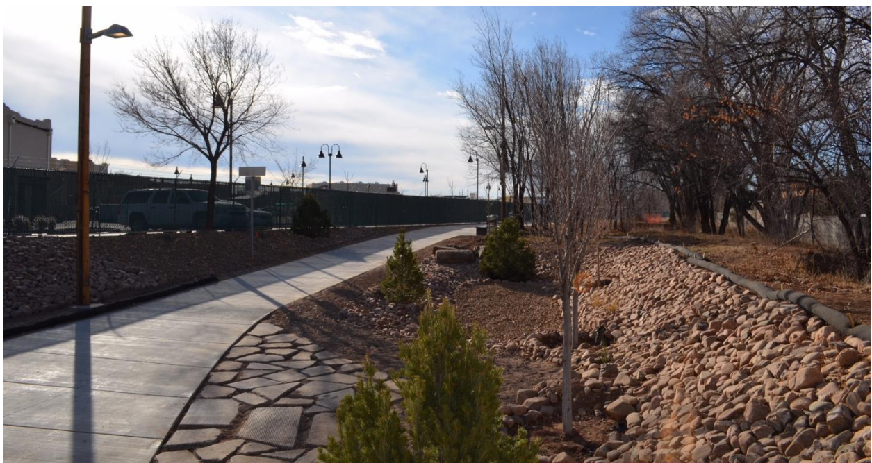
Figure 1. Acequia Underpass Bioretention
