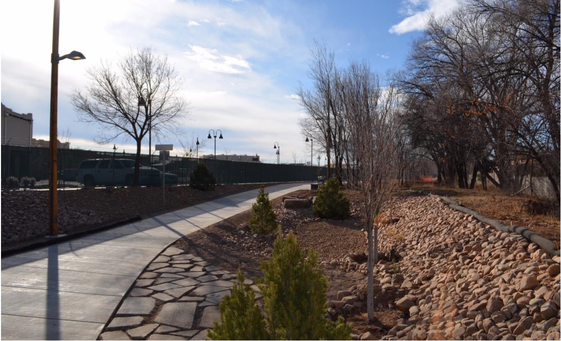
Example of a Bioretention Basin, Acequia Underpass (Photo Credit: Leroy Pacheco, City of Santa Fe)
