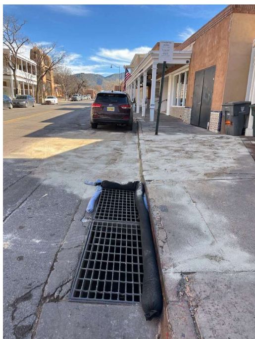
Illicit discharge mitigation from grease hood washing at a downtown restaurant.
