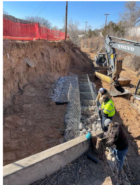
Construction of erosion control structures in an arroyo.
