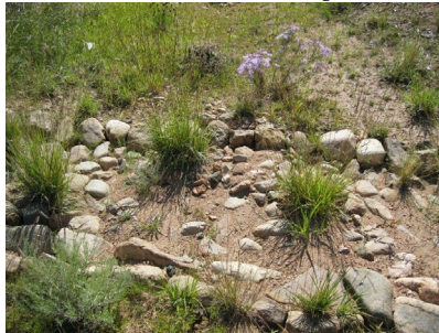
Open Channel Outfall – BMP – Infiltration Garden
