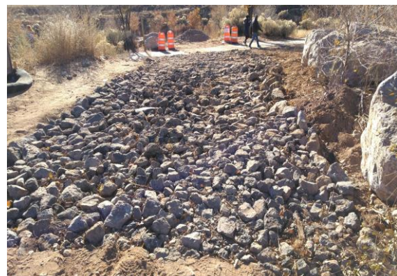
Photos 6 & 7: Protected Storm Drain and Track Pad Entrance at the 500C (CWSRF 088)-Santa Fe River Repair Project.
