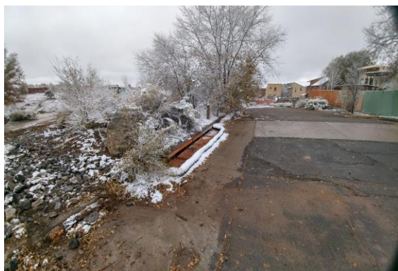
Photos 6 & 7: Protected Storm Drain and Track Pad Entrance at the 500C (CWSRF 088)-Santa Fe River Repair Project.
