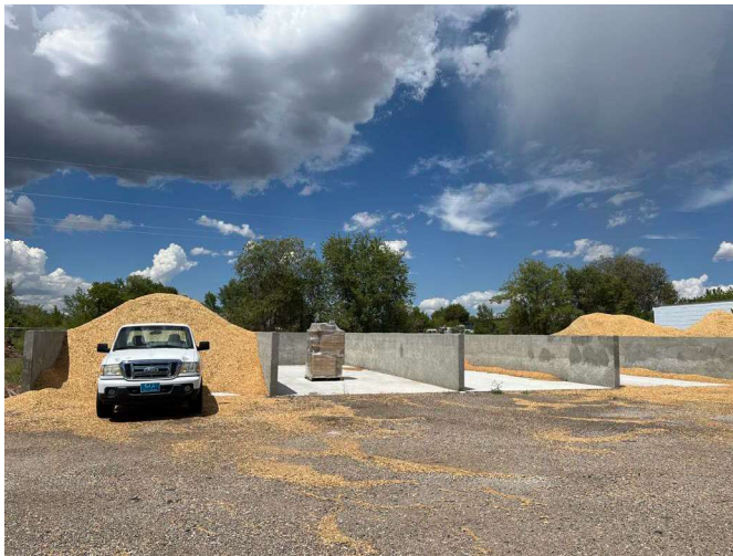
Newly built bays for mulch and other landscape materials to prevent wind and rain migration to storm system, Siler Yard Complex, 2024
