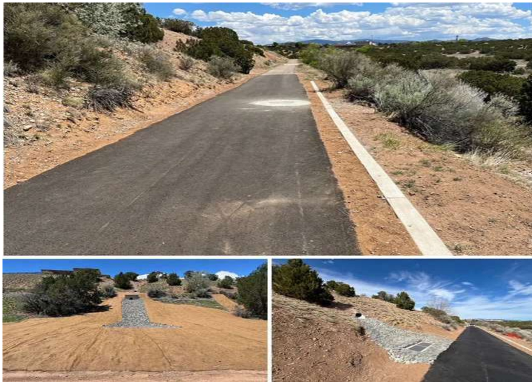
The Tierra Contenta Trail Repair to stop erosion and undermining of trail along the Arroyo de los Chamisos. 6/30/2024
