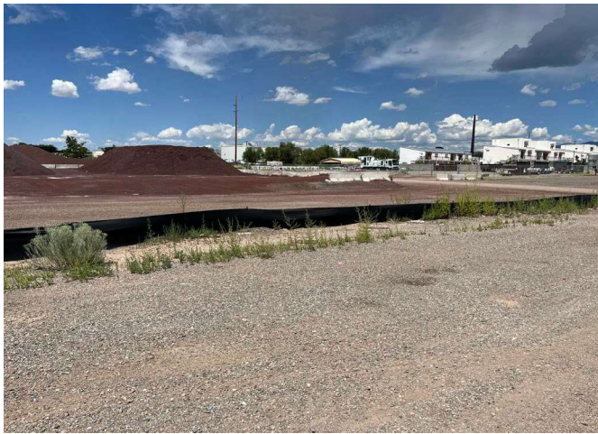
Silt fencing around salt and cinder yard prevents migration to the storm drain system, Siler Yard Complex 2024
