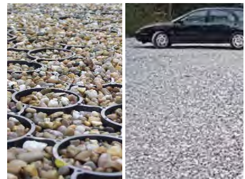
Permeable pavement used in a low-volume parking lot. Photos: Los Alamos National Laboratory, 2017
