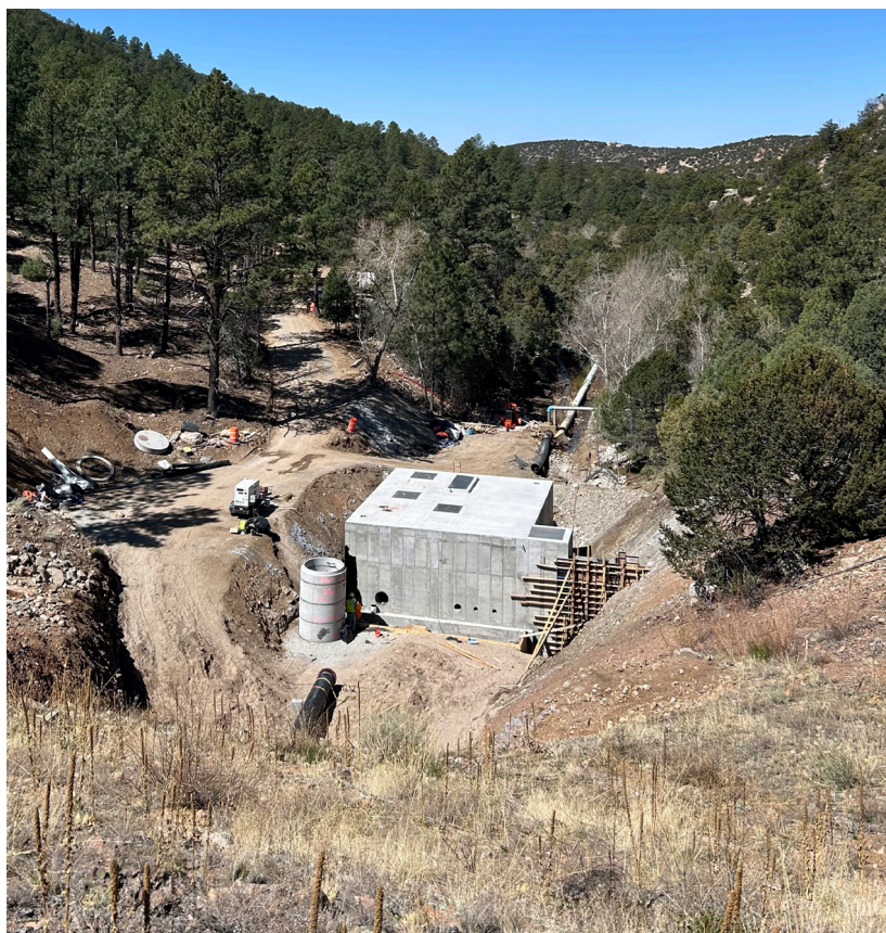
35 – Construction of the new Nichols valve vault
