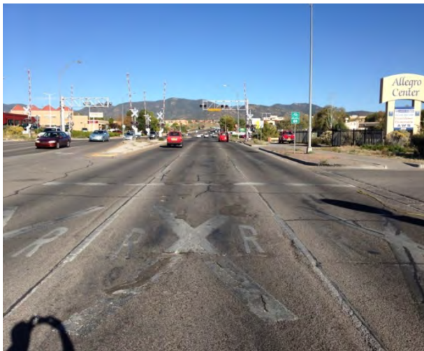
Eastbound St. Michael's Drive Approaching NMRX Crossing
