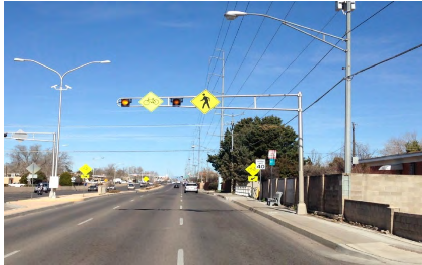
Figure 4.8 Type II Mastarm with Flashers and Pedestrian/Bicycle Signage
