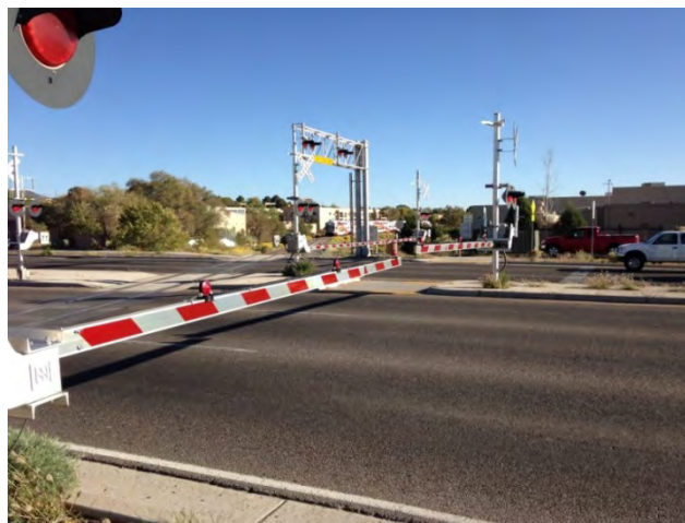
Figure 2.5 St. Michael's Drive Rail Crossing Traffic Control
