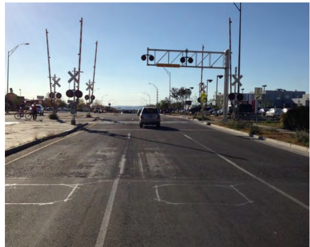
Westbound St. Michael's Drive Approaching NMRX Crossing
