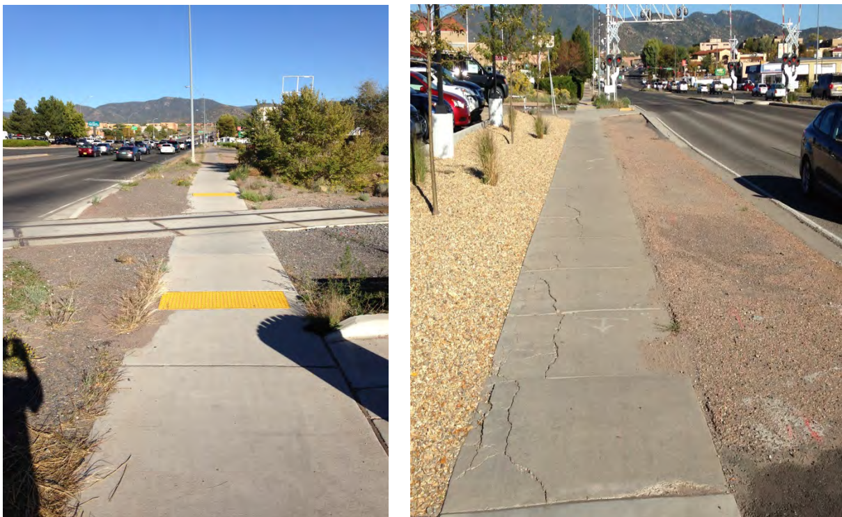
Figure 2.6 Pedestrian Facilities along St. Michael's Drive at Santa Fe Rail Trail
