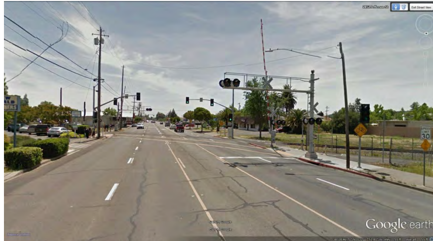
Figure 4.7 Southbound Jefferson Street approaching Napa Wine Train Crossing
