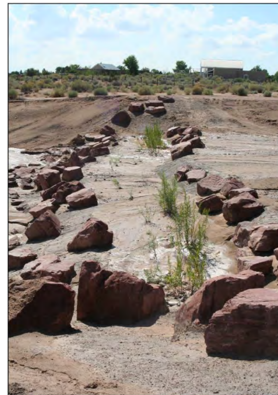
Photograph: Grade control structure in the Lower Montoyas arroyo incorporating planting strip. (Source: SSCAFCA)
