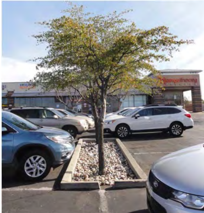
Curb inlets to tree trench pavilions in parking lot in Albuquerque, NM (2)
