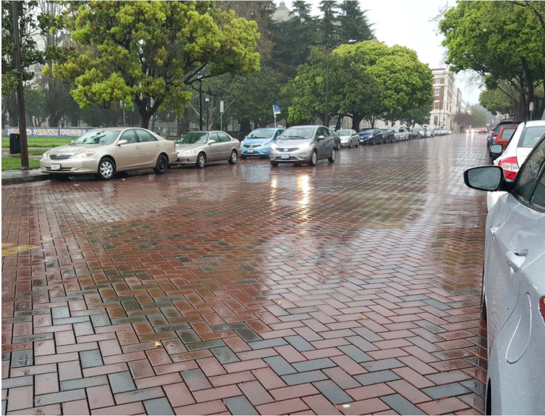
Allston Way in Berkeley, California was completely renovated with permeable interlocking concrete pavers. (Photo Source: https://www.cleanwaterprogram.org/index.php/programs/green-infrastructure/greenstreets-examples.html )
