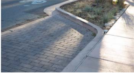
Urban example of permeable pavement (1)
