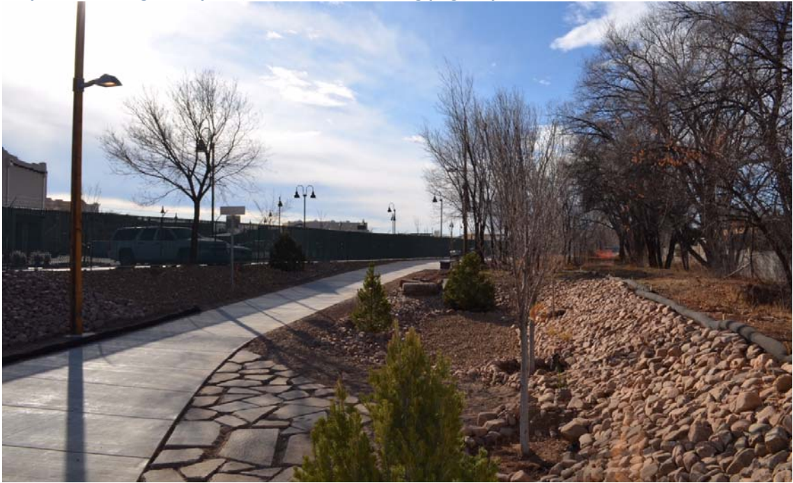
Example of a Bioretention Basin, Acequia Underpass (Photo Credit: Leroy Pacheco, City of Santa Fe)
