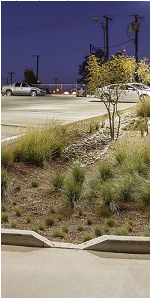
Example of a bioswale with bioretention/bioinfiltration taking stormwater from a parking Lot (2)
