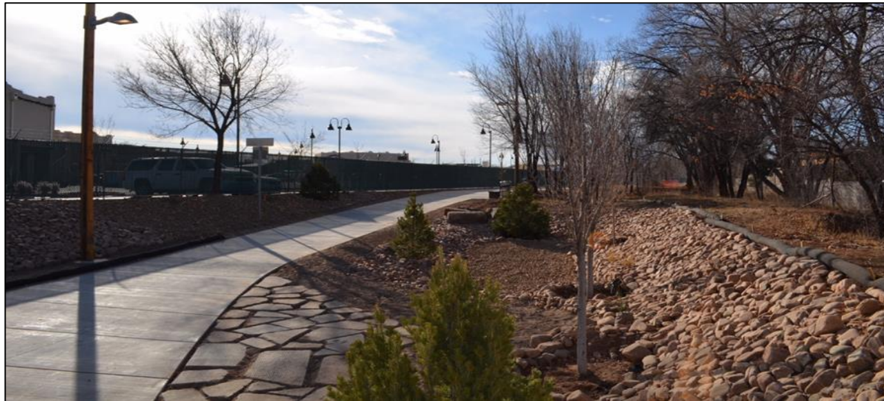
Photograph: Stormwater swale installed as a component of the Acequia Trail Underpass project (Source: City of Santa Fe)
