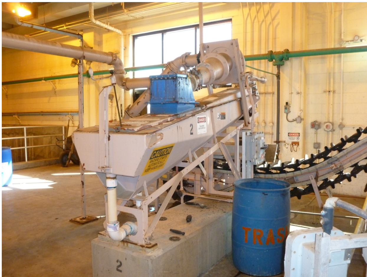
Figure 8-2. Picture of the Existing Grit Classifier Equipment
