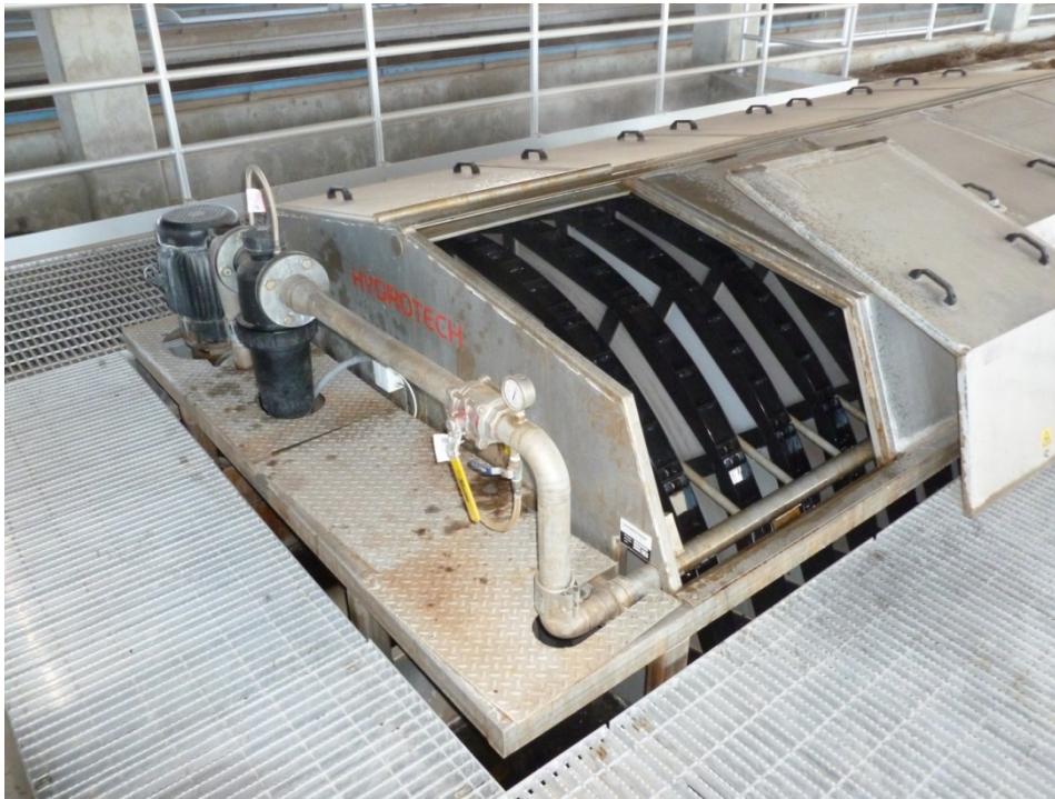
Figure 8-6. Picture of the Existing Disk Filtration Equipment
