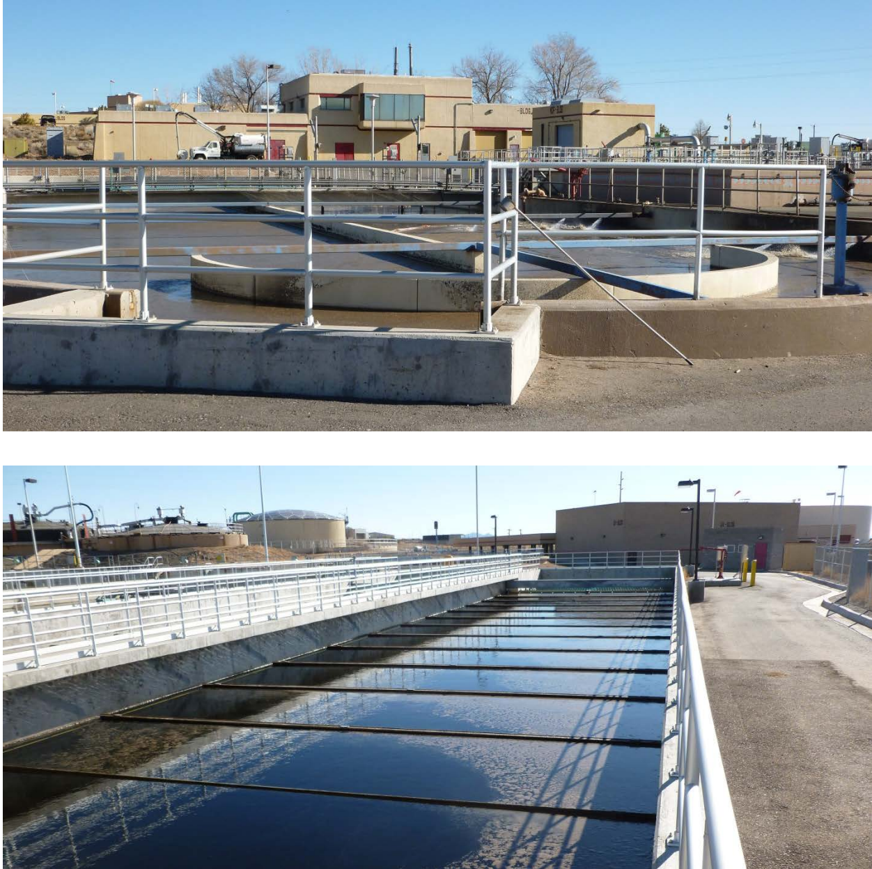
Figure 8-4. Picture of the Existing Aeration Basins (Top) and Final Clarifiers (Bottom)
