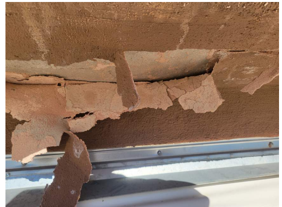
Damaged stucco | A9
