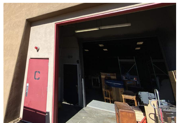
Roll door and hollow metal door | A7
