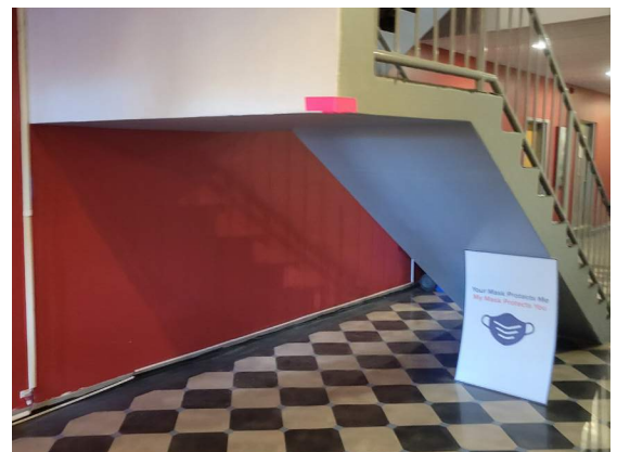
Unprotected area under stair | A31
