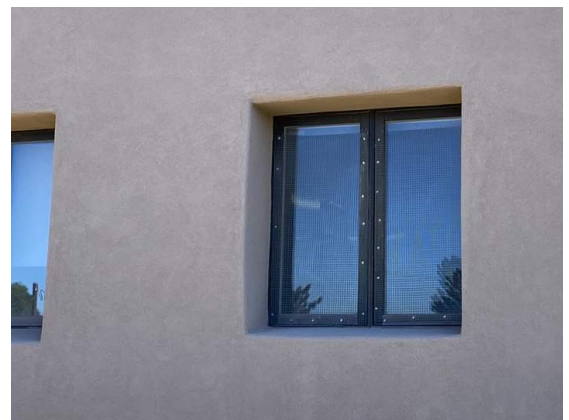
Window covered with wire mesh | A6
