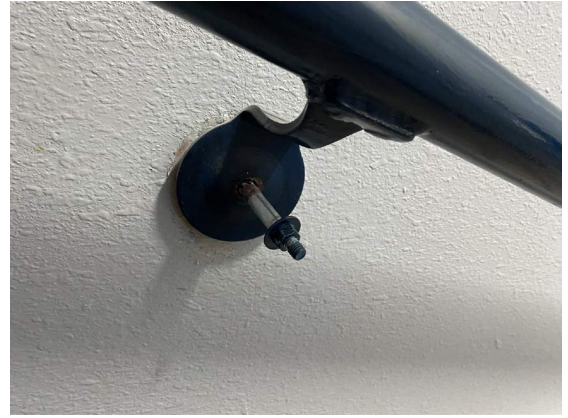
Handrail bolt falling out | A16
