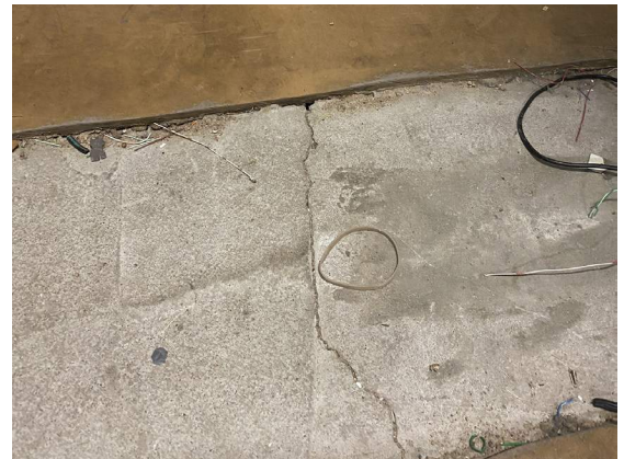
Patched floor in electrical room | A29
