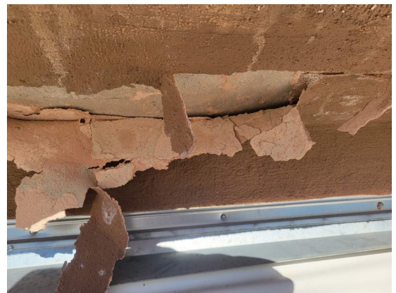
Stucco damage on the roof | A30
