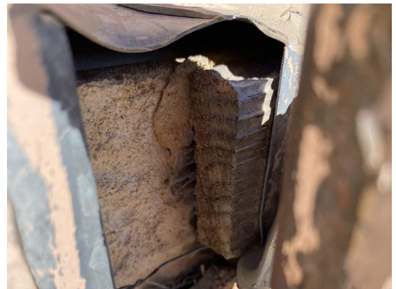
Stucco and flashing damage | A31
