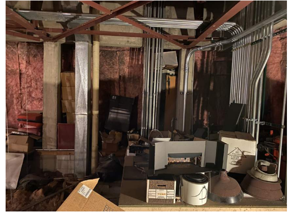
Example of attic contents | A16
