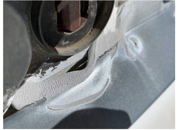
Metal flashing at roof membrane edge | A8
