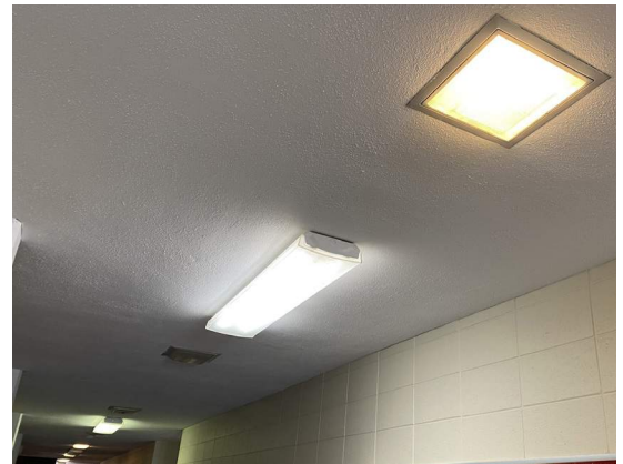
Mixed light fixtures in hallway | A29
