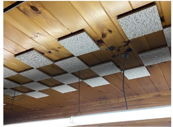
Acoustic tile adhered to wood ceiling | A12
