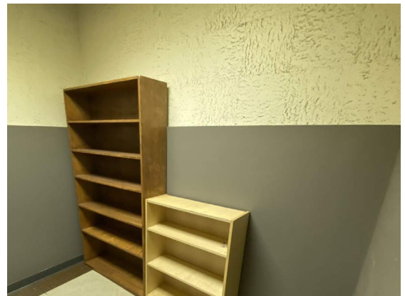
Acoustic tiles adhered to CMU | A11
