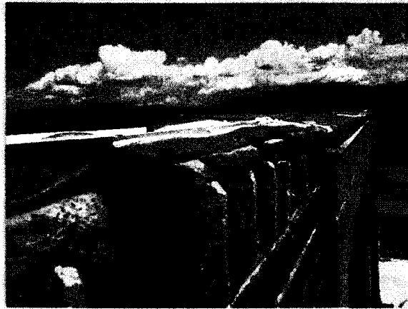
Photo 14- Brick and Mortar Deterioration at Top of South Wall.
