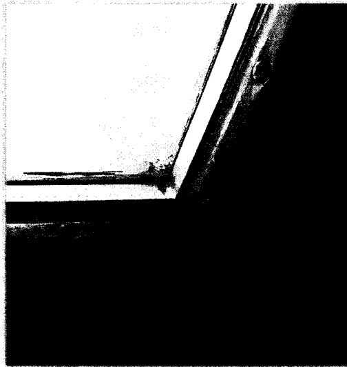
Photo 28-Corrosion at hollow metal windows
