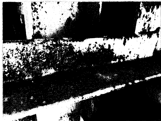
Photo 7- Corrosion on Bottom Chord of Truss
