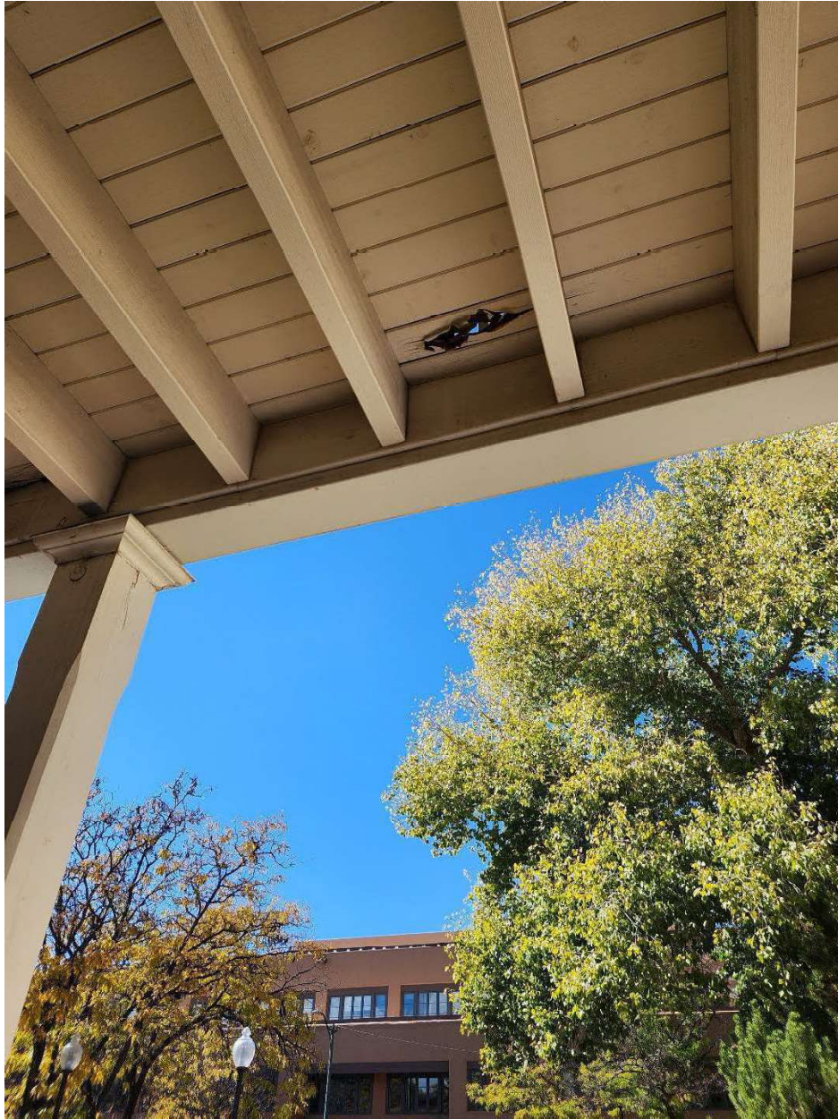
Example of deteriorating woodwork to the point of disintegration.
