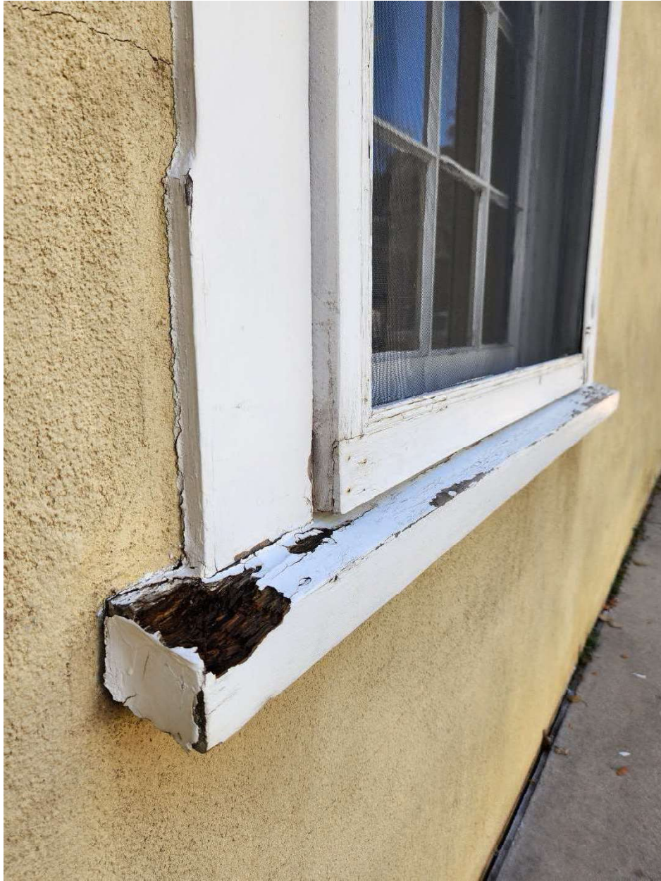
Example of deterioration to point of disintegration.
