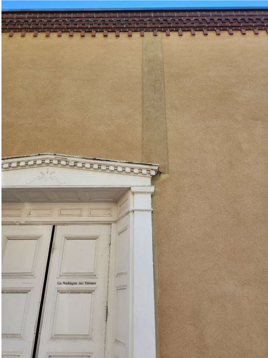
Example of stucco deterioration.
