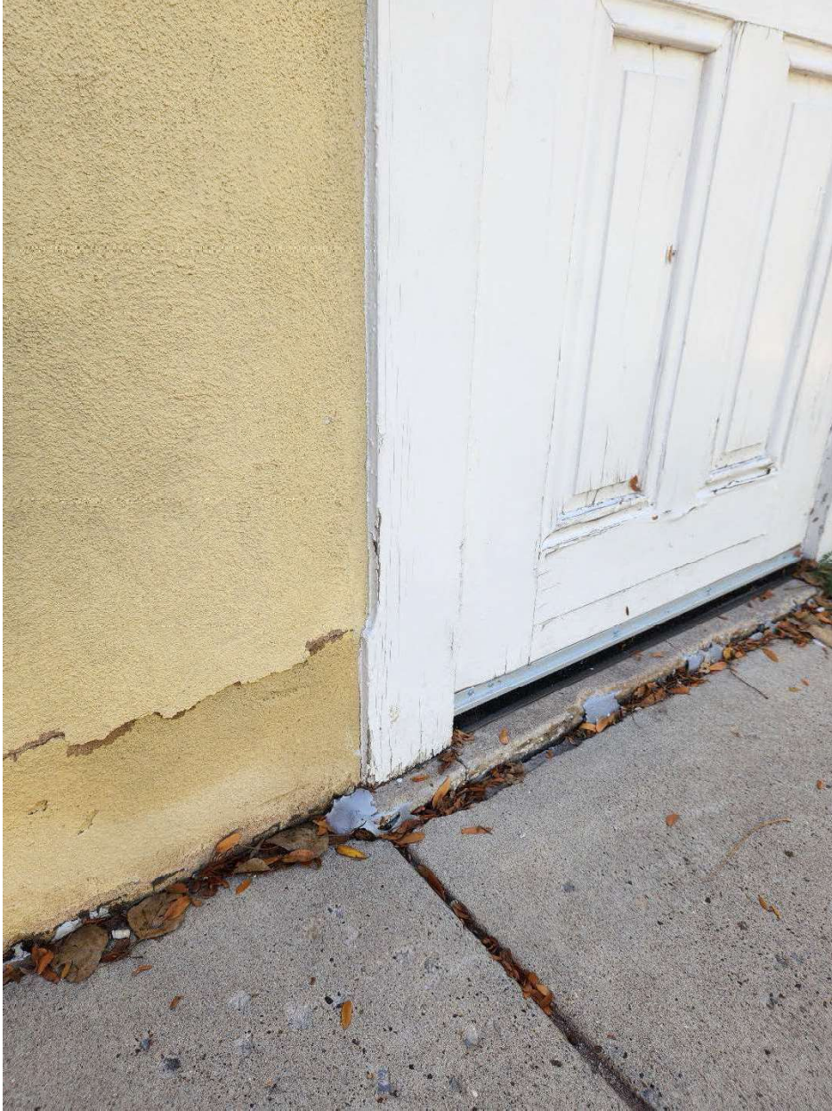
Example of deterioration and apparent settlement of wall and stucco.
