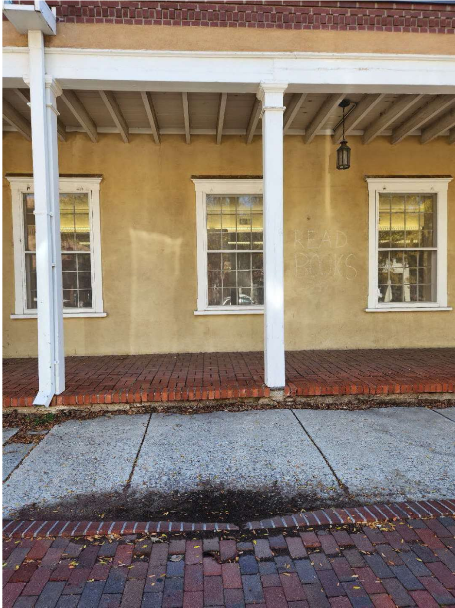
Examples of paving, woodwork, and stucco deterioration.
