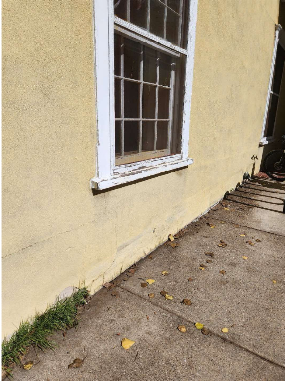
Example of stucco deterioration.
