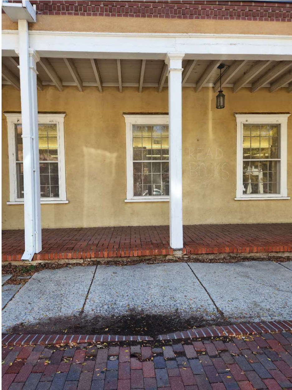
Examples of paving, woodwork, and stucco deterioration.
