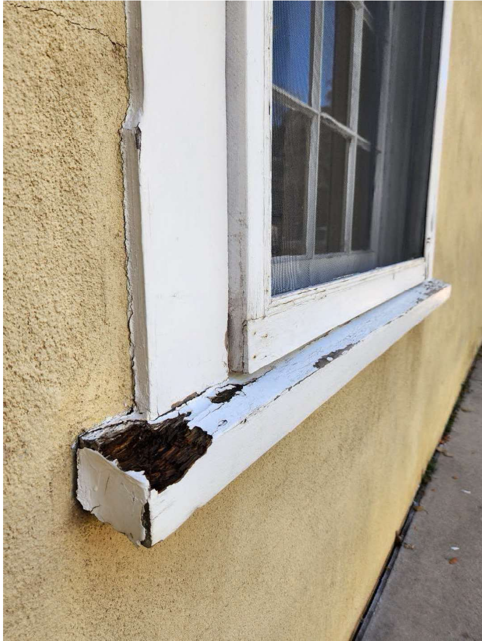
Example of deterioration to point of disintegration.
