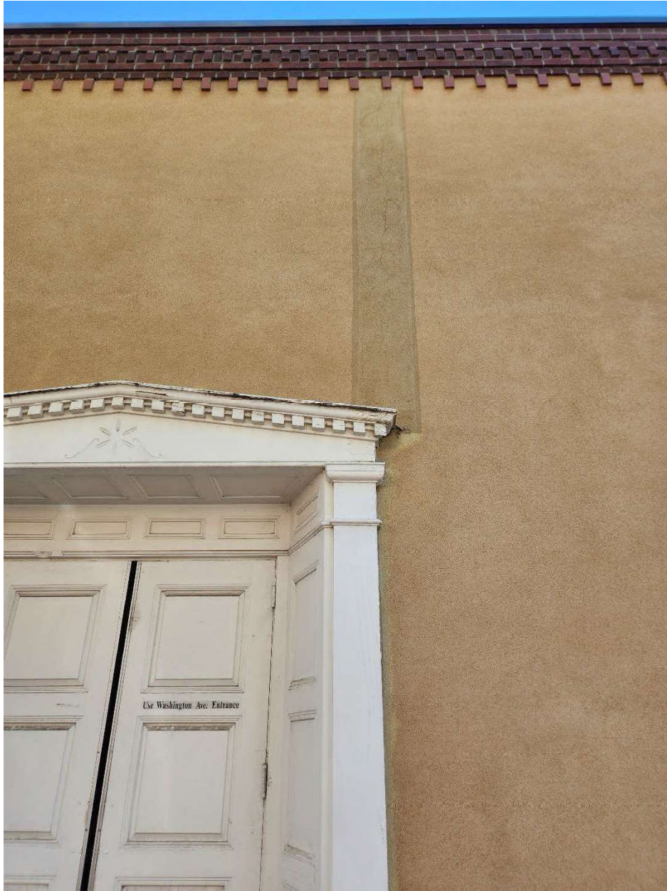
Example of stucco deterioration.
