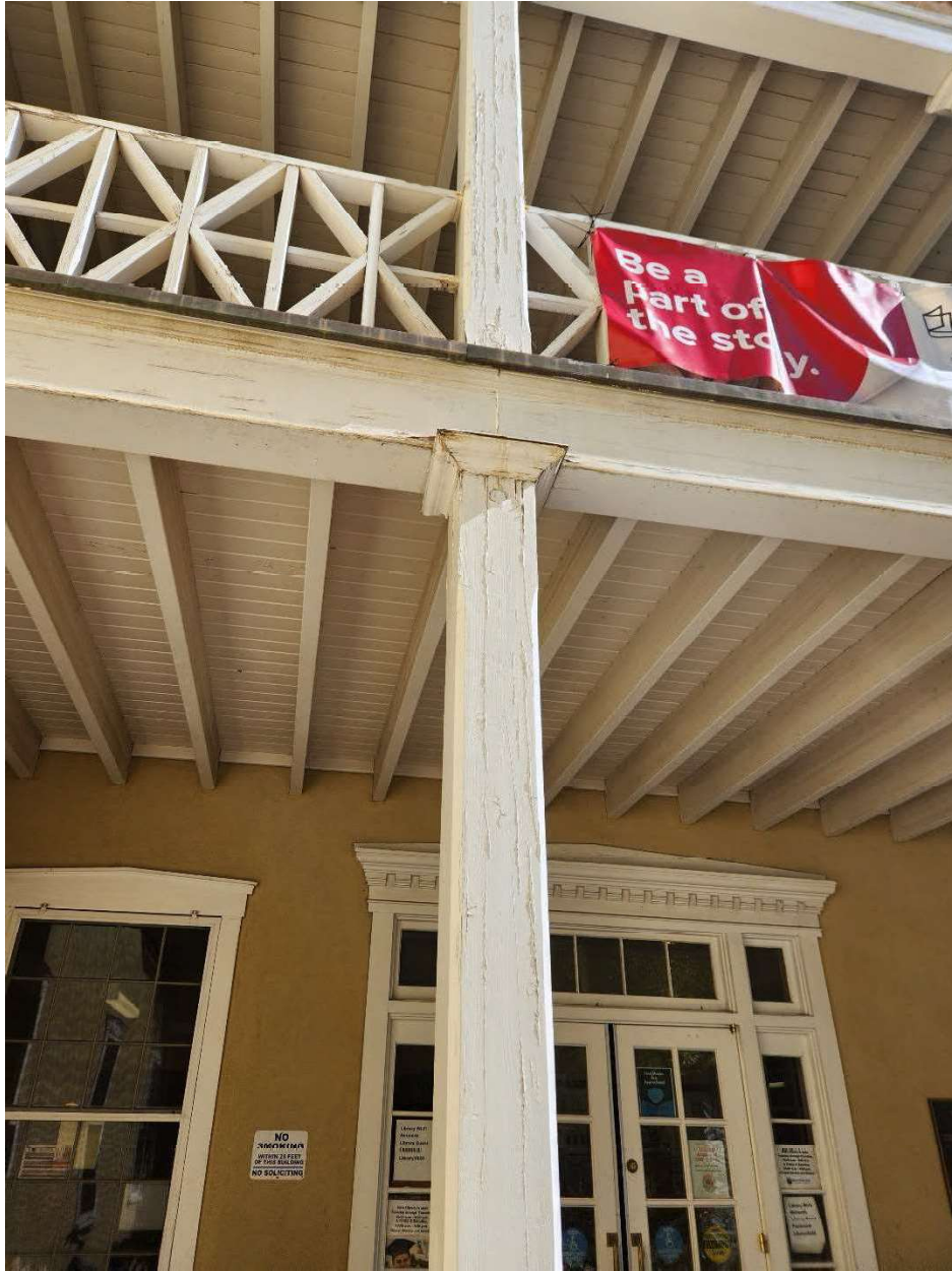
Examples of deteriorating woodwork .
