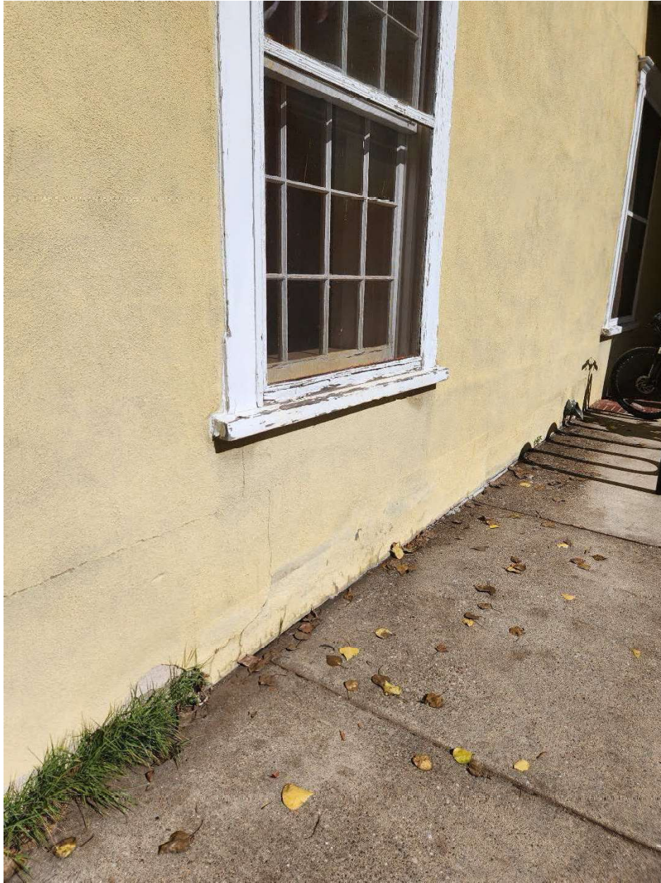
Example of stucco deterioration.
